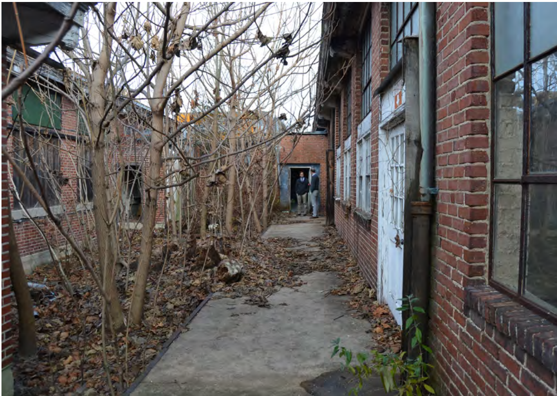
96. Grey Mill, Courtyard, Looking North
