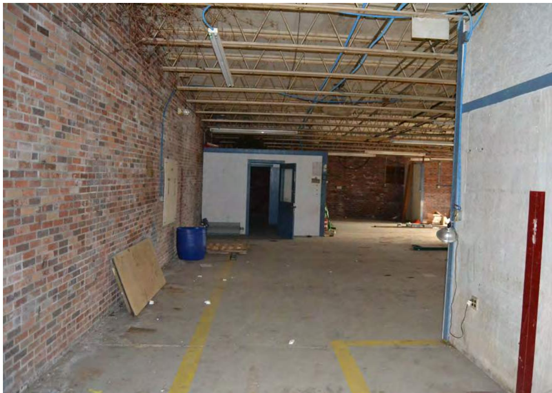
87. Grey Mill, 1970s Warehouse, Looking East
