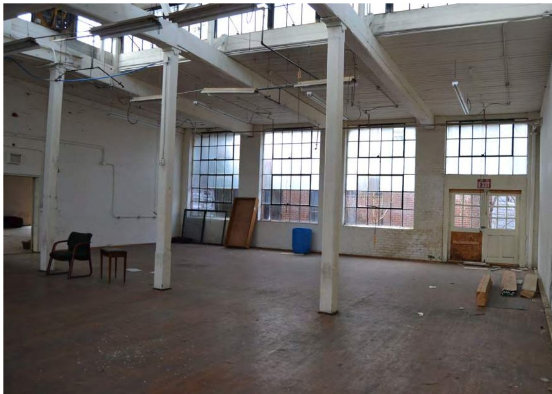
70. Grey Mill, 1926 Addition, Finishing Room, Looking Southwest
