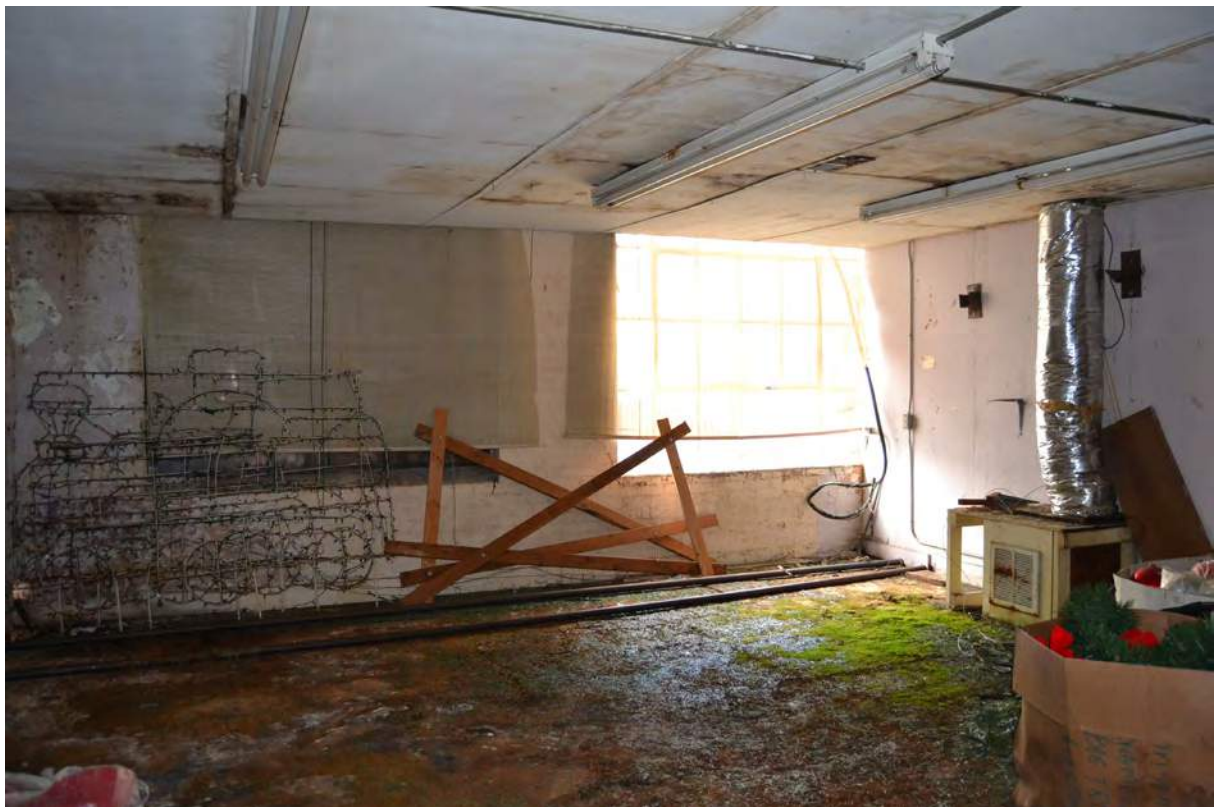
38. Grey Mill, 1915 Building, Looking West
