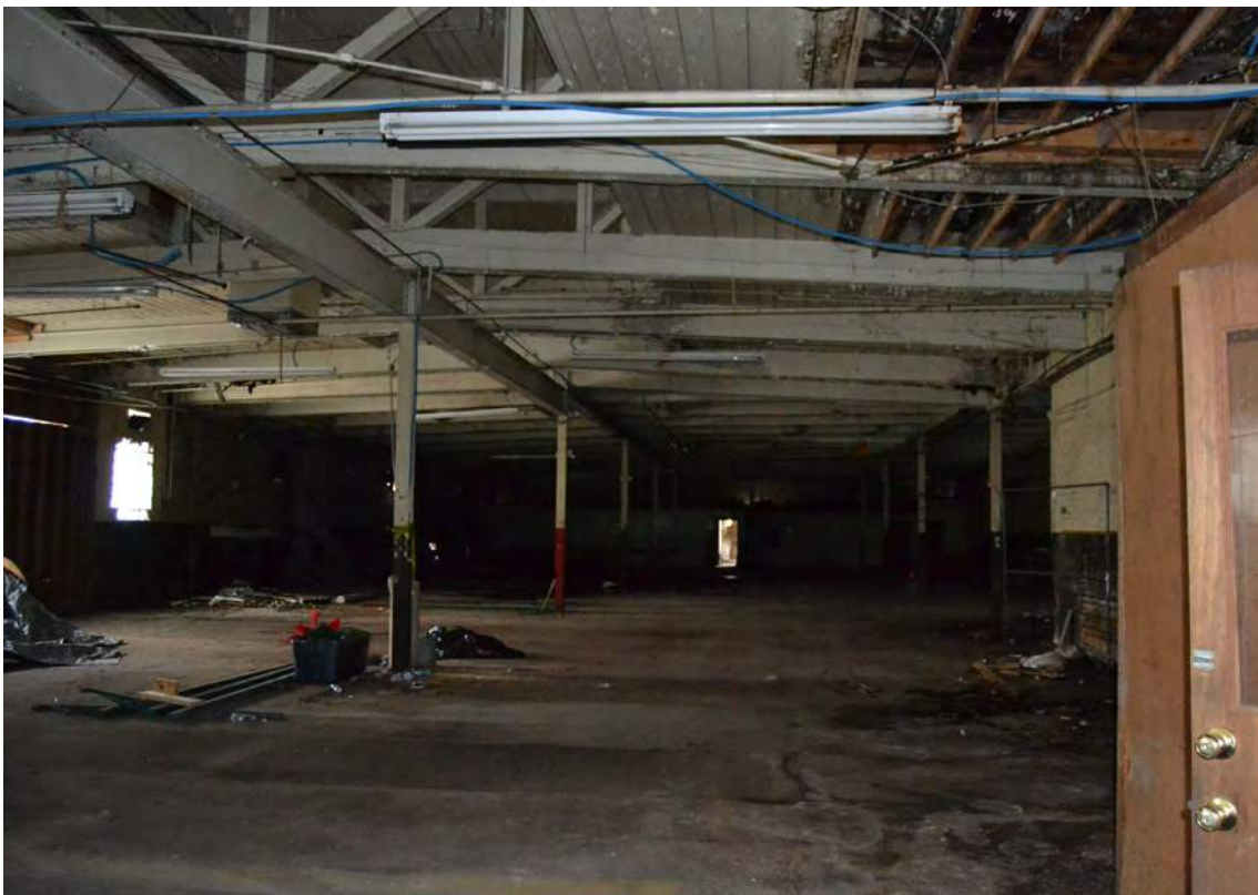
44. Grey Mill, 1947 Addition, Looking North
