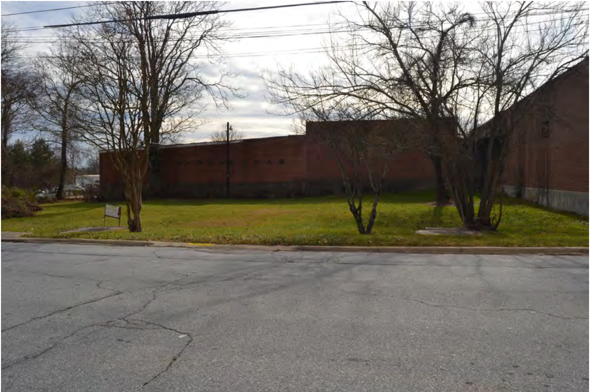
15. Grey Mill, 1947 Addition, North Elevation, Looking South
