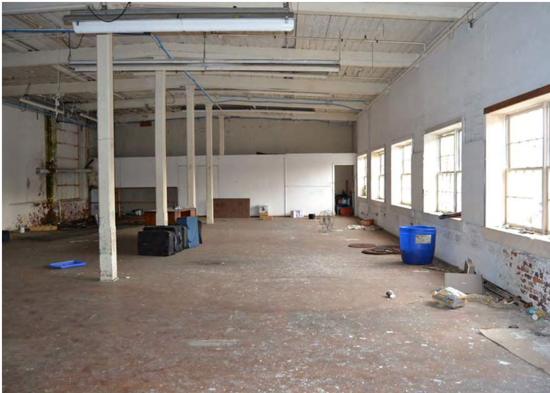
55. Grey Mill, 1919 Building, Looking East
