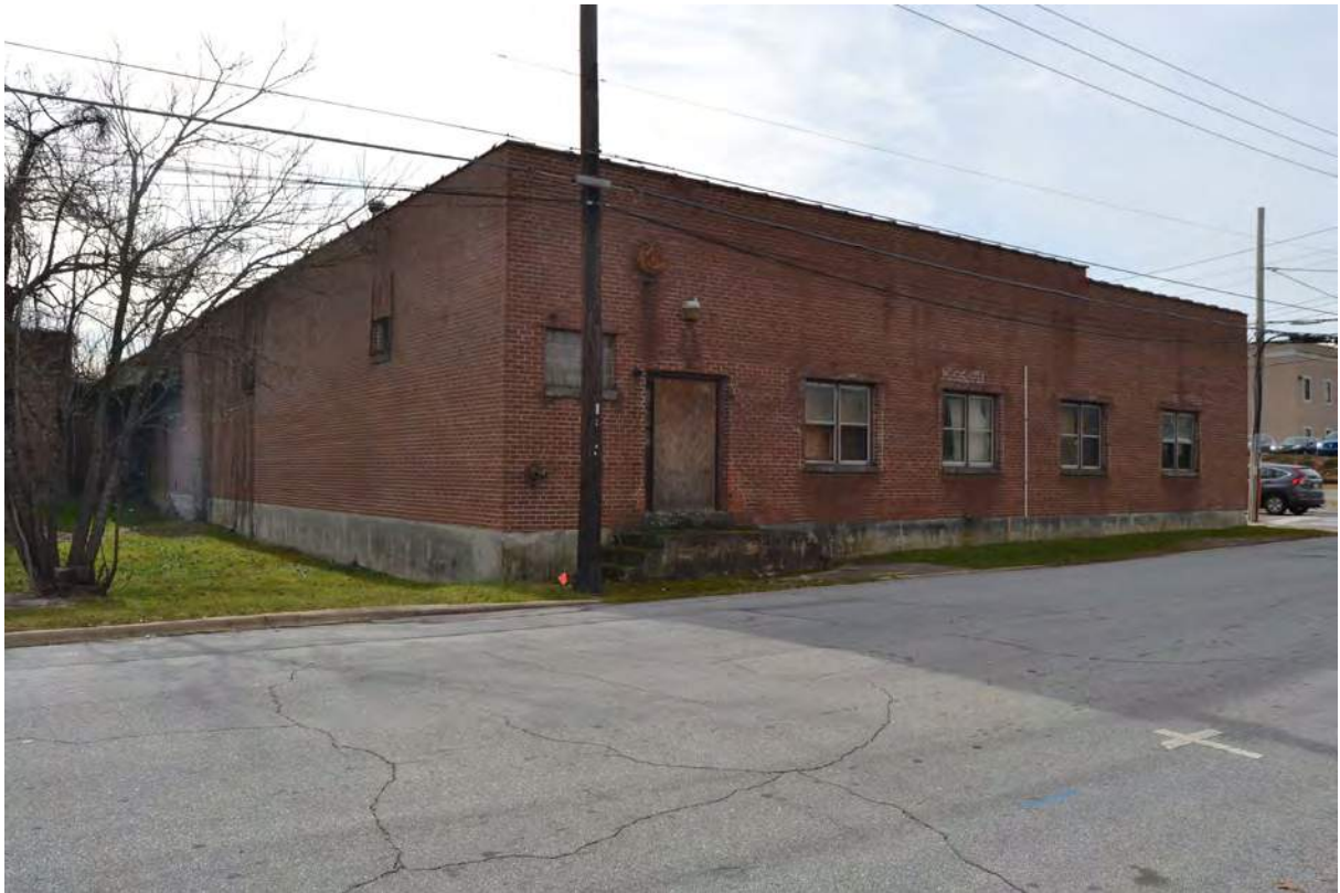
13. Grey Mill, 1947 Addition, North Elevation, Looking Southwest
