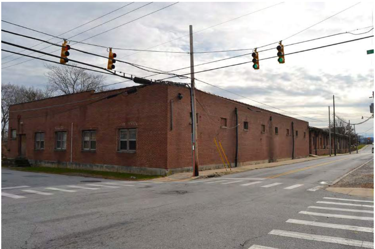
12. Grey Mill, 1947 Addition, Northwest Corner, Looking Southeast
