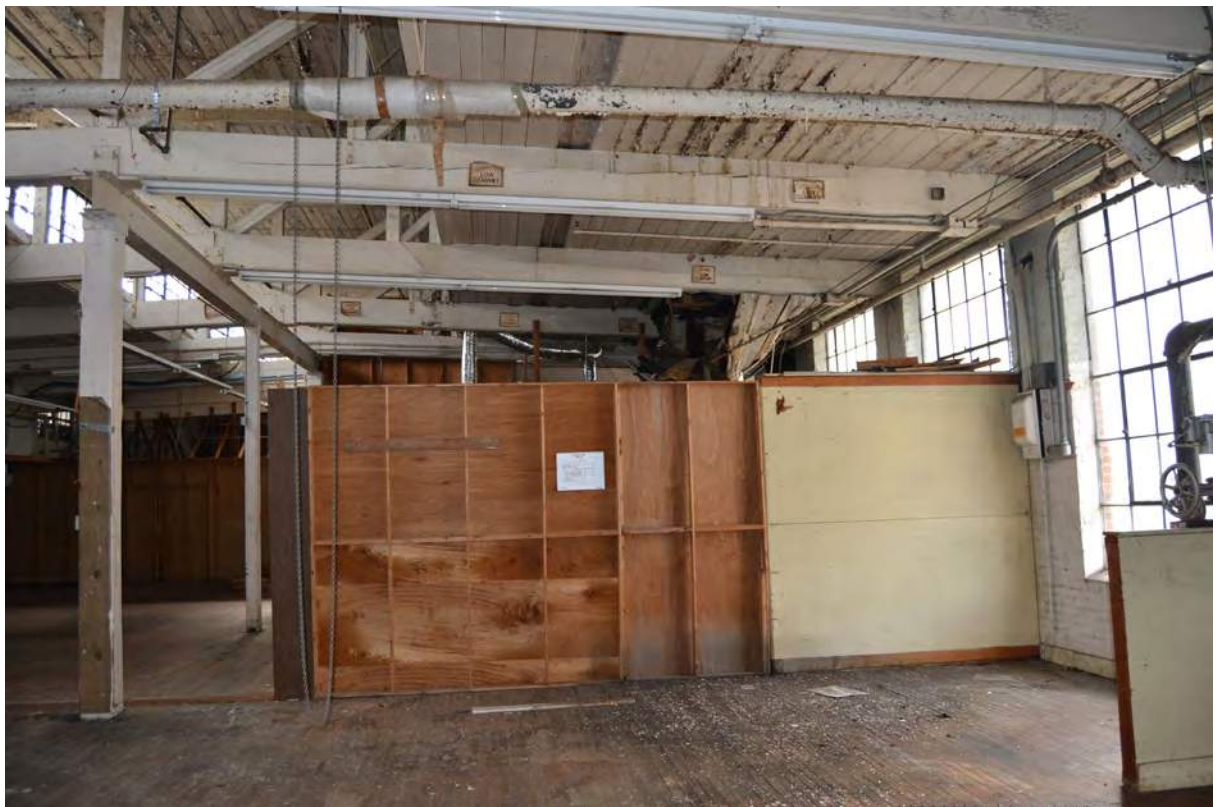
42. Grey Mill, 1915 Building, Looking South
