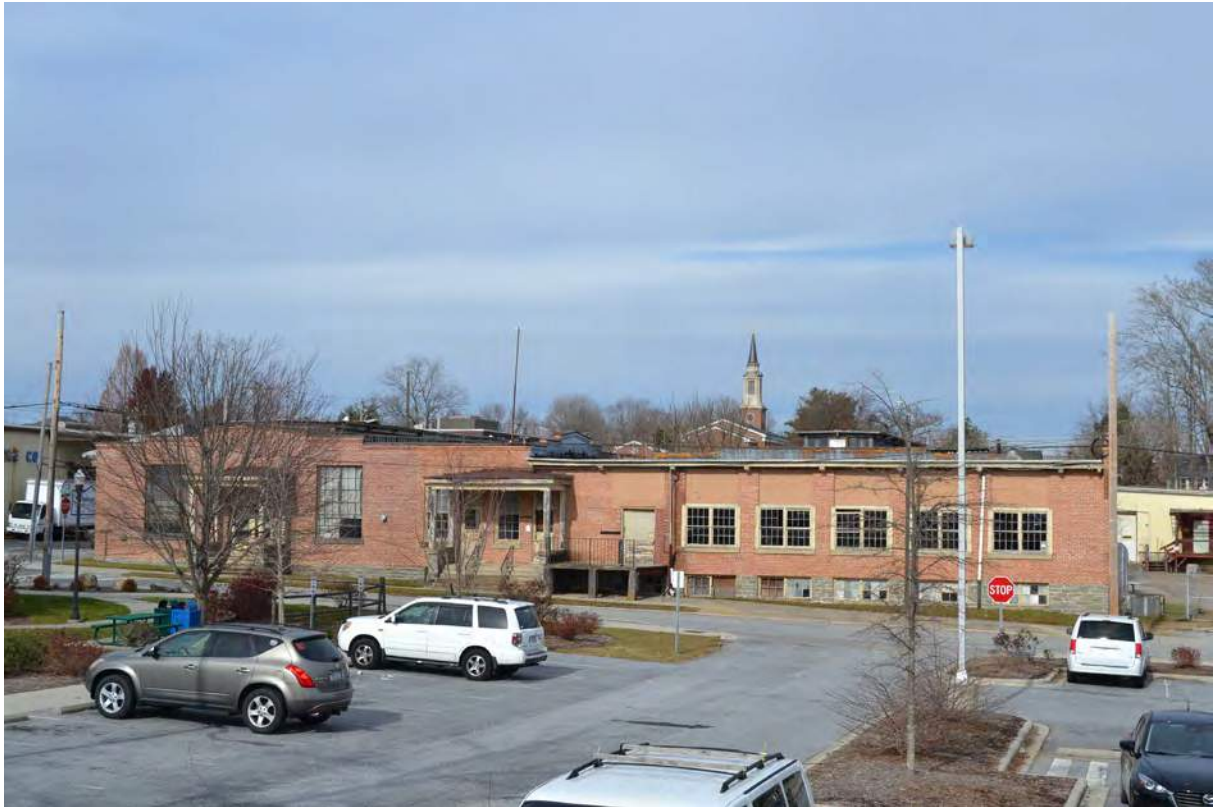
1. Grey Mill, South Facade, Looking North
