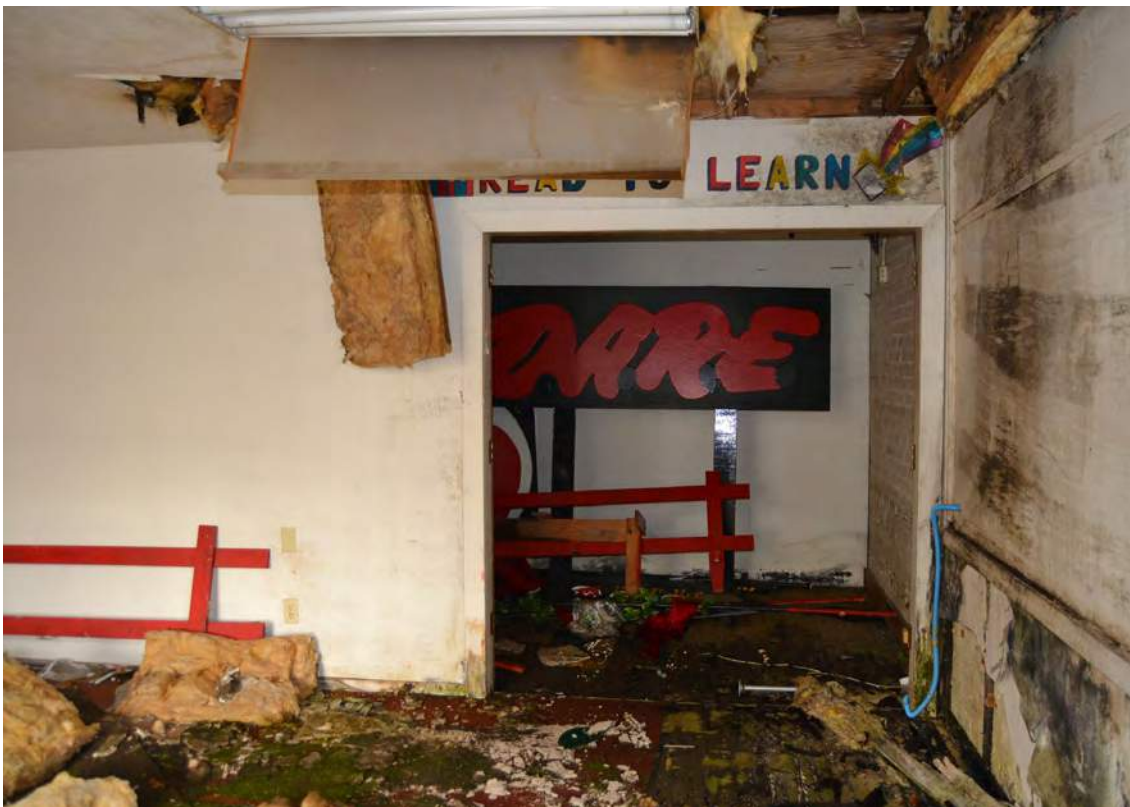
32. Grey Mill, 1915 Building, South End, Looking North
