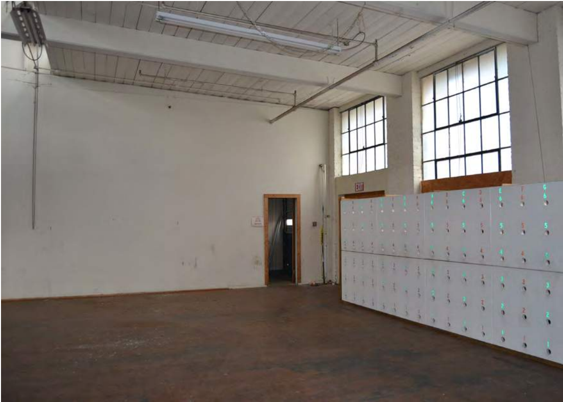
67. Grey Mill, 1926 Addition, Finishing Room, Looking Northeast
