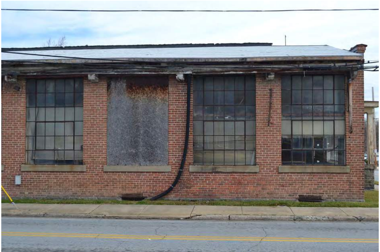
7. Grey Mill, 1915 Building, West Elevation, Window Detail
