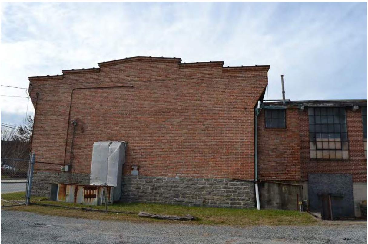
24. Grey Mill, 1919 Building, East Elevation, Looking West
