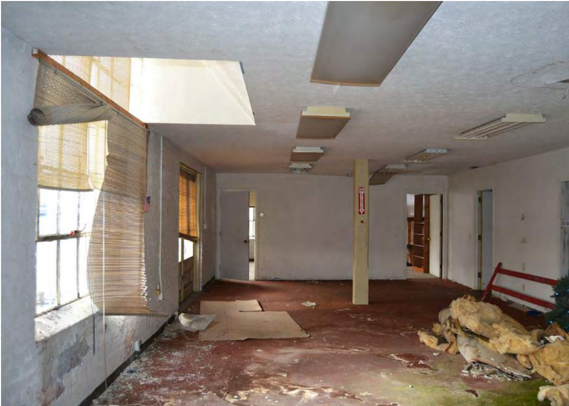
31. Grey Mill, 1915 Building, South End, Looking West
