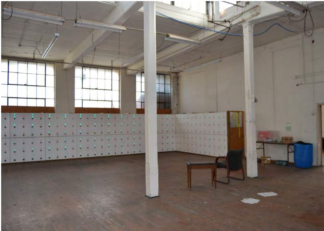
69. Grey Mill, 1926 Addition, Finishing Room, Looking Southeast
