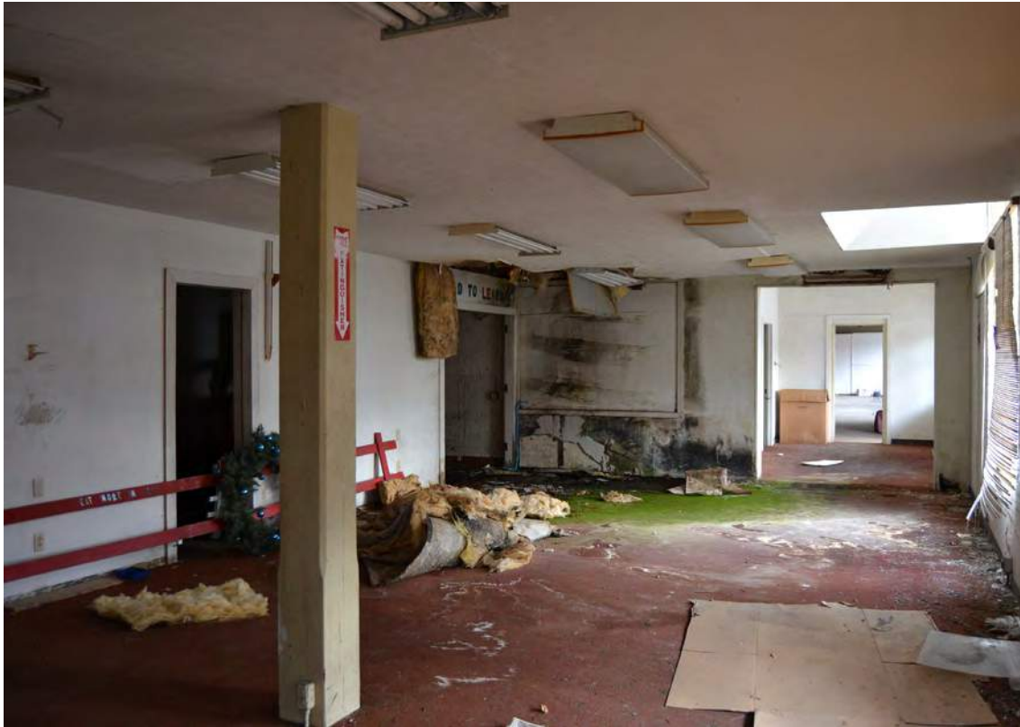
33. Grey Mill, 1915 Building, South End, Looking East
