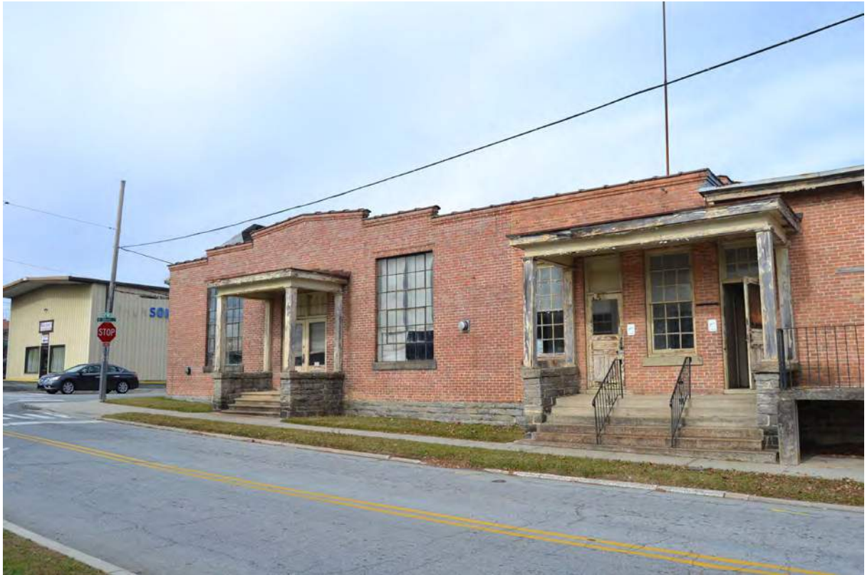
3. Grey Mill, 1915 Building, South Facade, Looking Northwest
