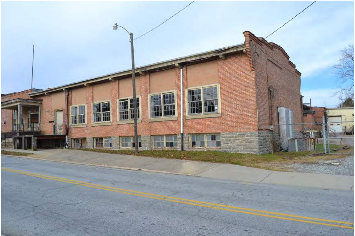
5. Grey Mill, 1919 Building, South Facade, Looking Northwest
