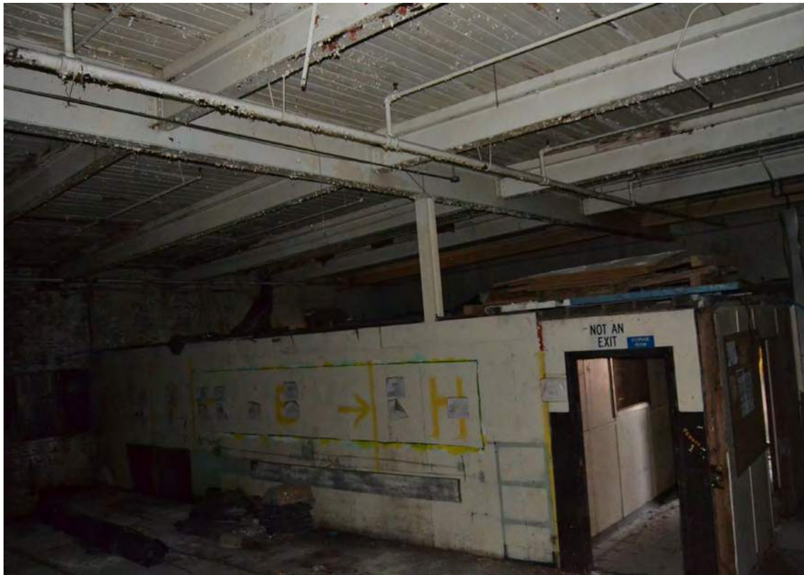
51. Grey Mill, 1947 Addition, Looking Northwest
