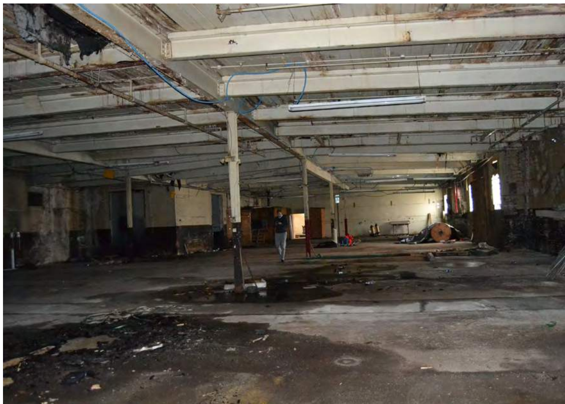
48. Grey Mill, 1947 Addition, Looking South
