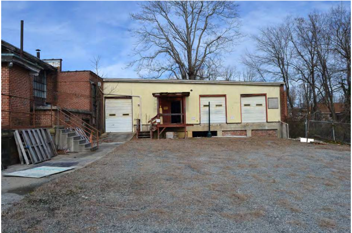
17. Grey Mill, 1970s Warehouse, Looking North
