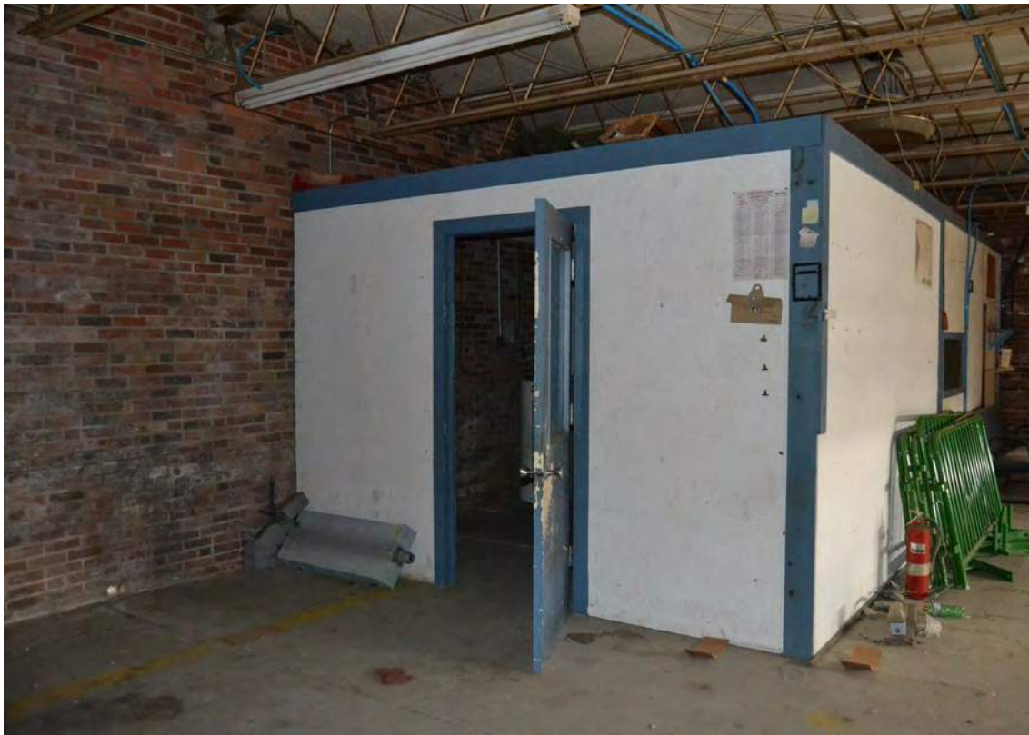
88. Grey Mill, 1970s Warehouse, Looking Northeast
