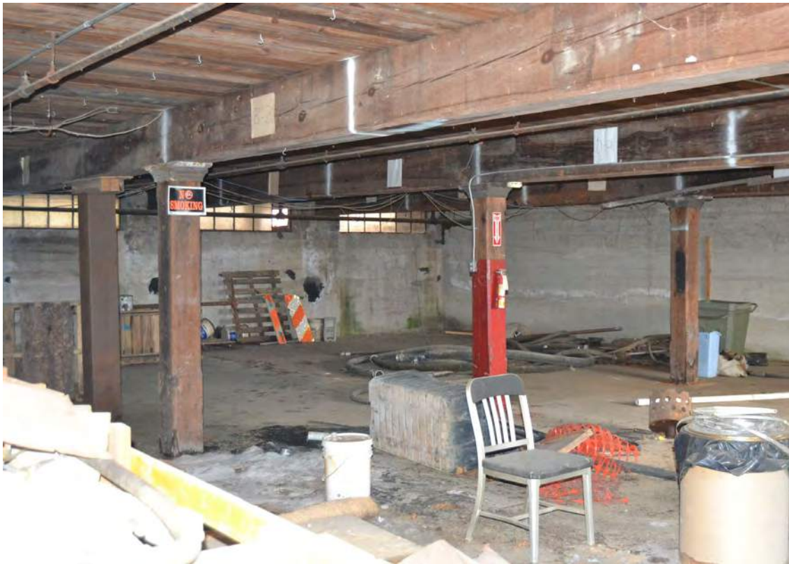
116. Grey Mill, Dye House Basement, Looking Northwest
