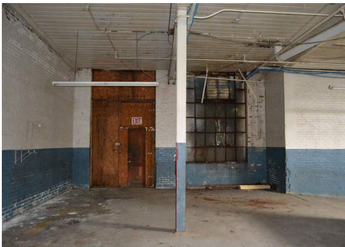
81. Grey Mill, 1926 Addition, Looking East
