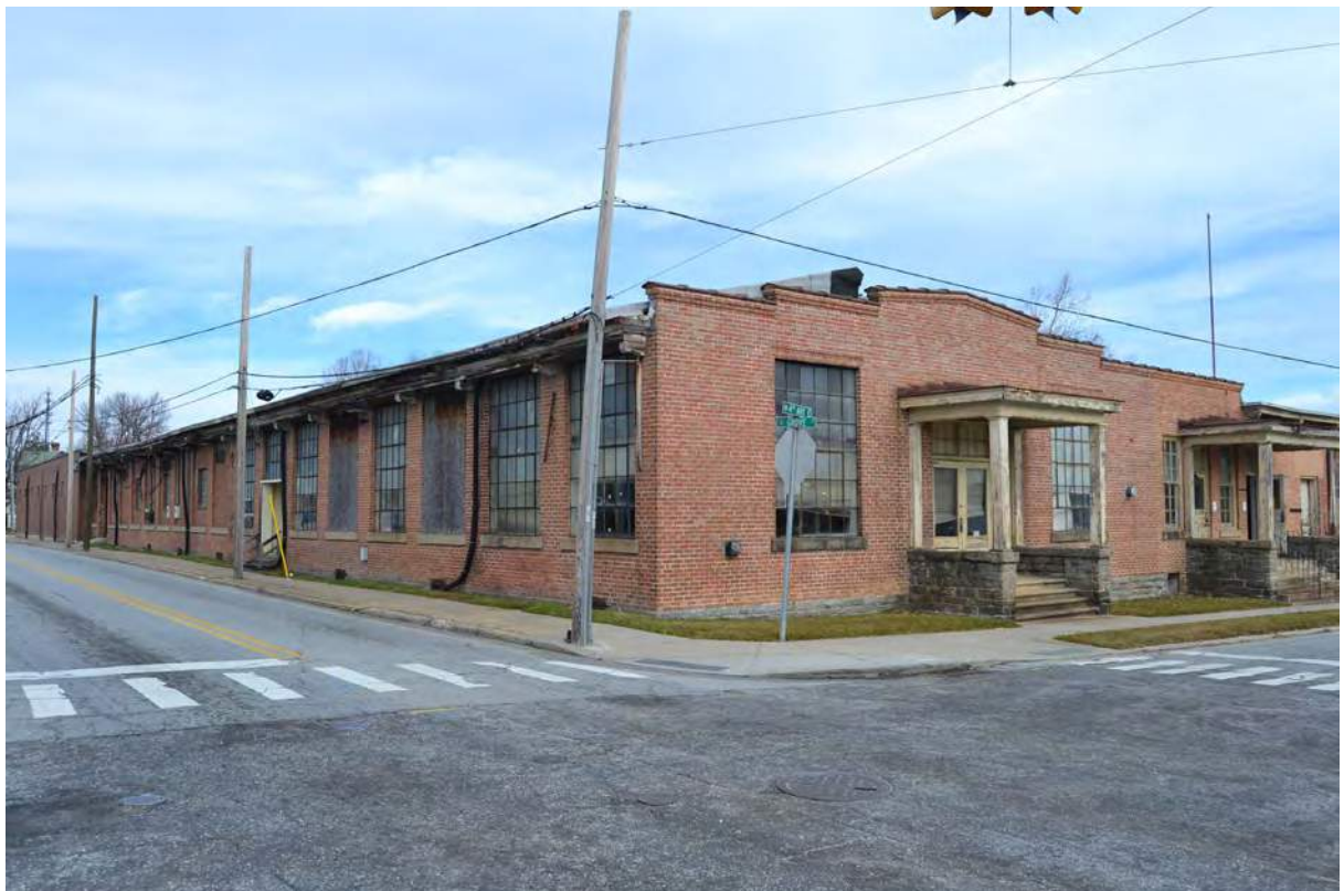
2. Grey Mill, 1915 Building, Southwest Corner, Looking Northeast
