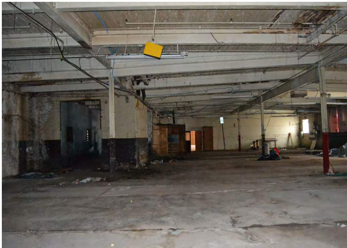
52. Grey Mill, 1947 Addition, Looking South
