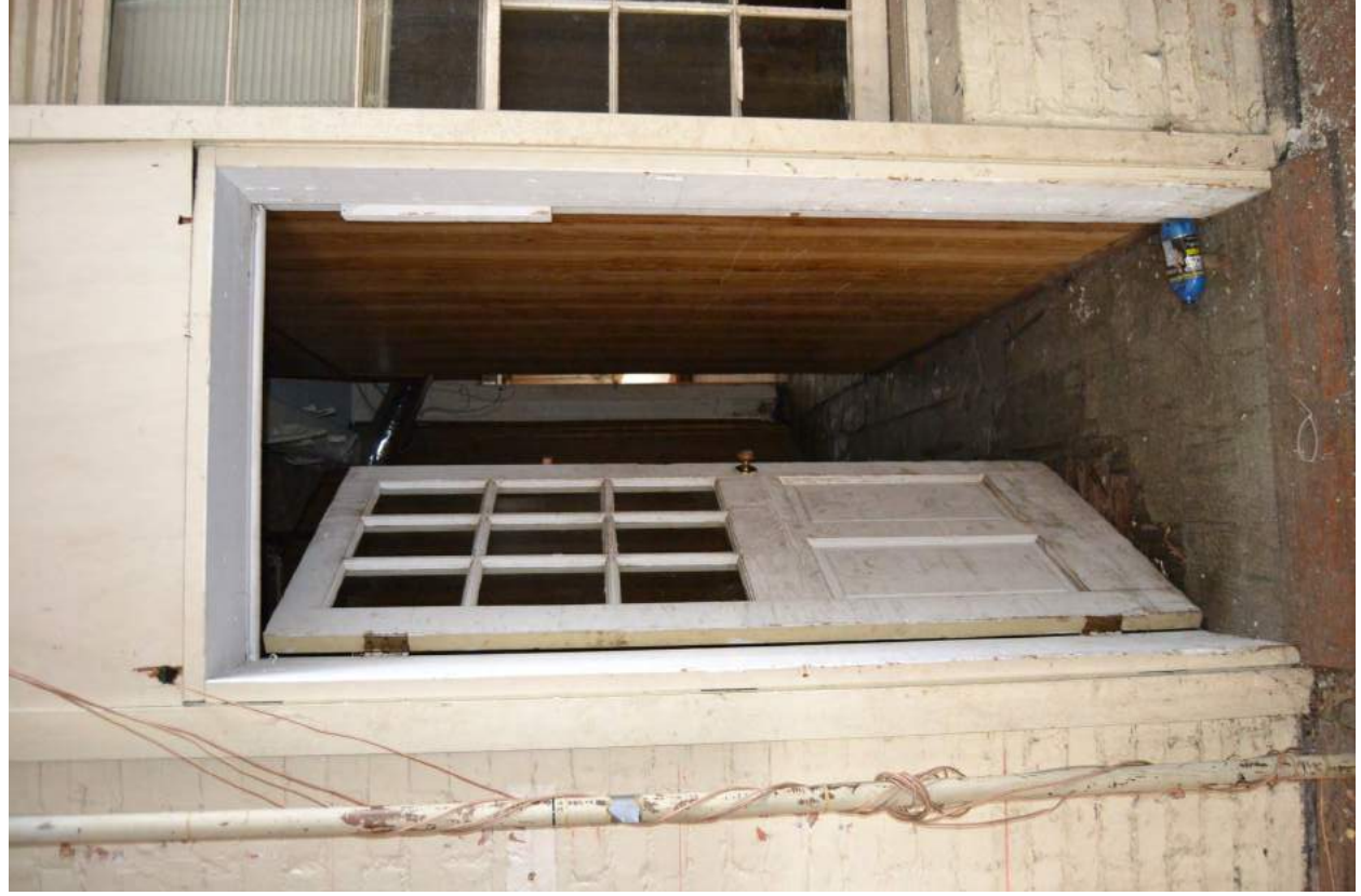
28. Grey Mill, Rear Office, Looking West
