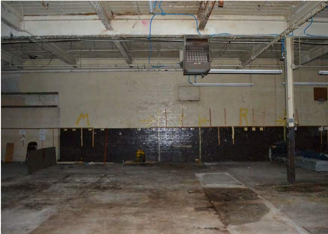
49. Grey Mill, 1947 Addition, Looking East
