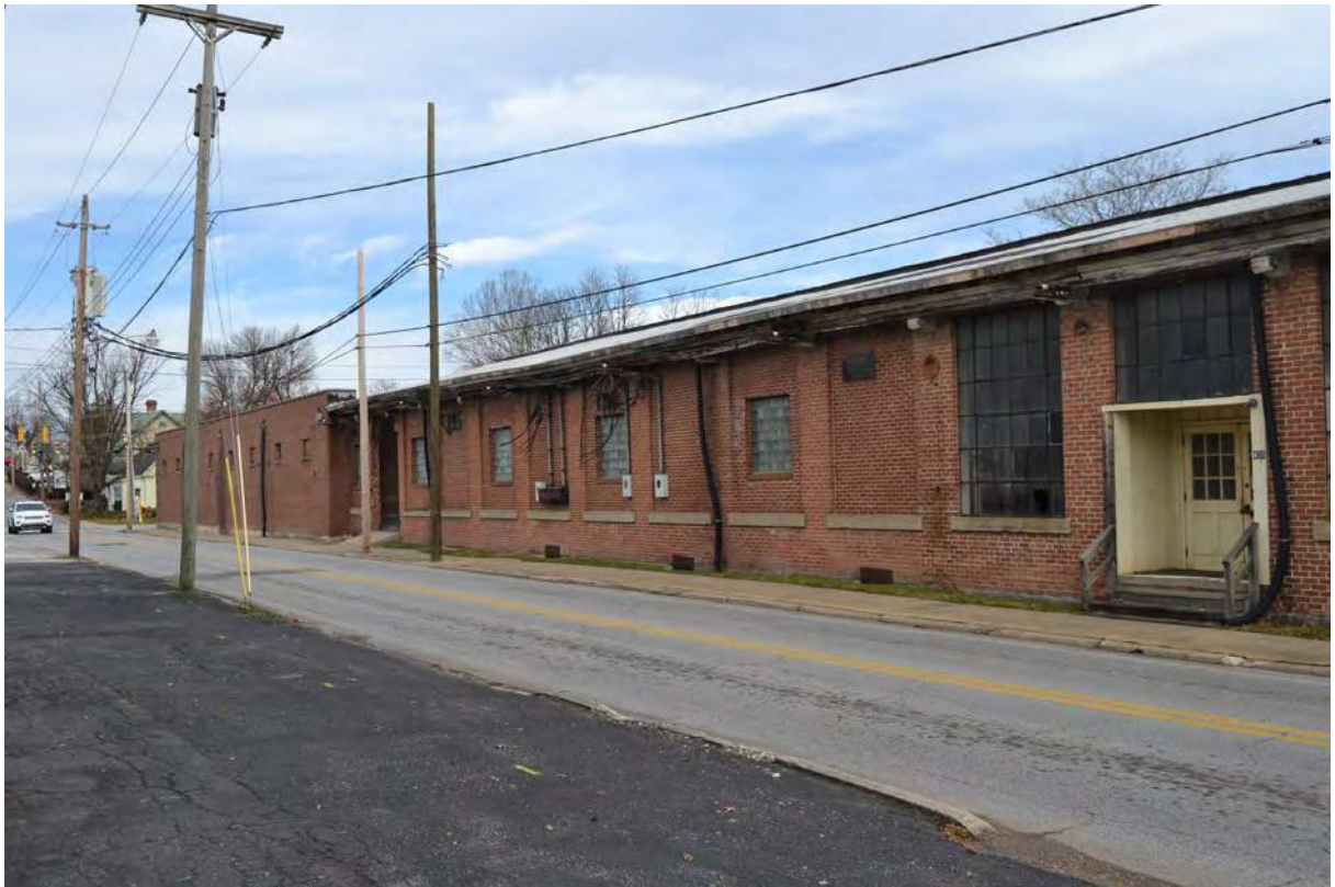
9. Grey Mill, 1915 Building, West Elevation, Looking Northeast
