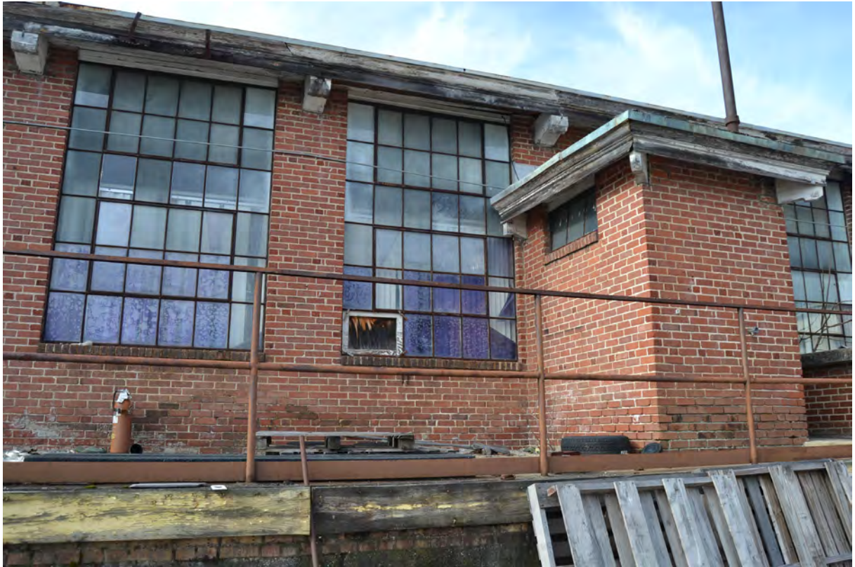
21. Grey Mill, 1919 Building, East Elevation, Window Detail
