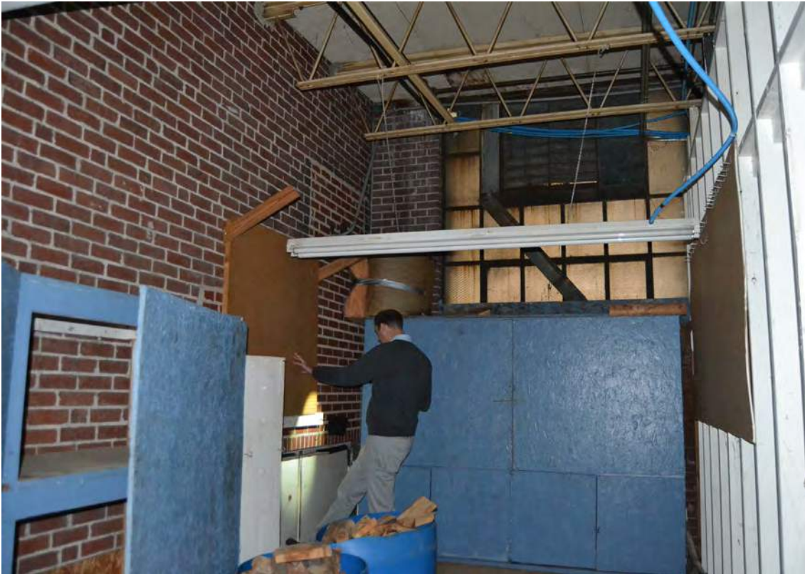
90. Grey Mill, 1970s Warehouse, Looking West
