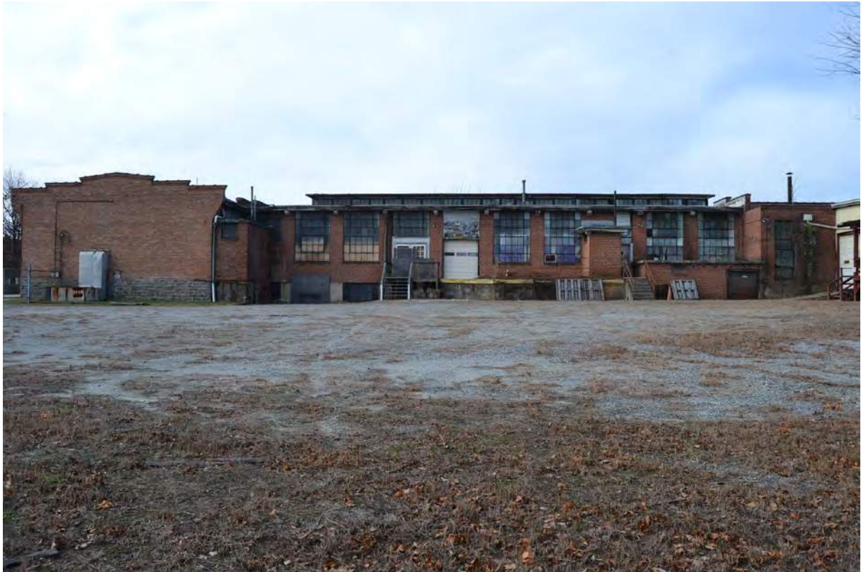
19. Grey Mill, 1919 Building, East Elevation, Looking West
