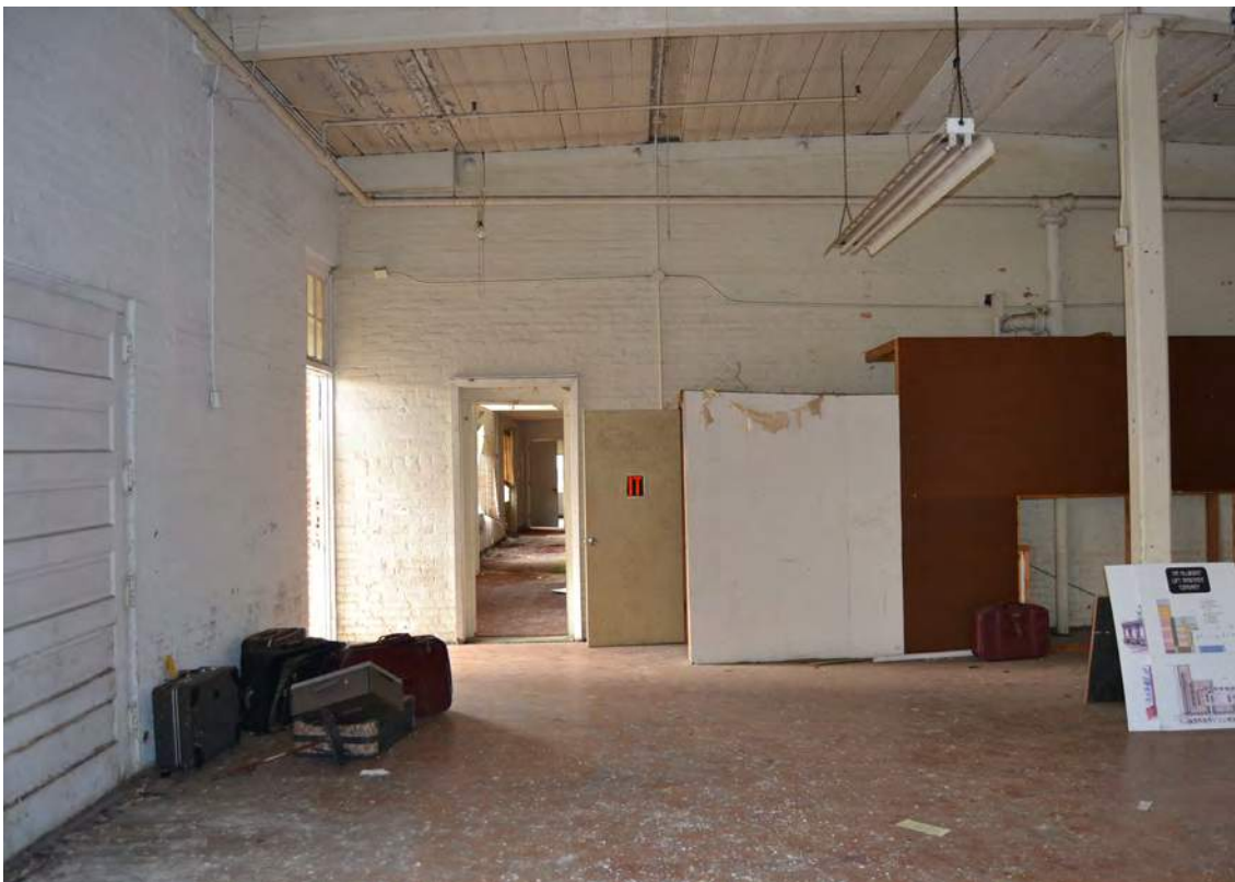
64. Grey Mill, 1919 Building, Looking West
