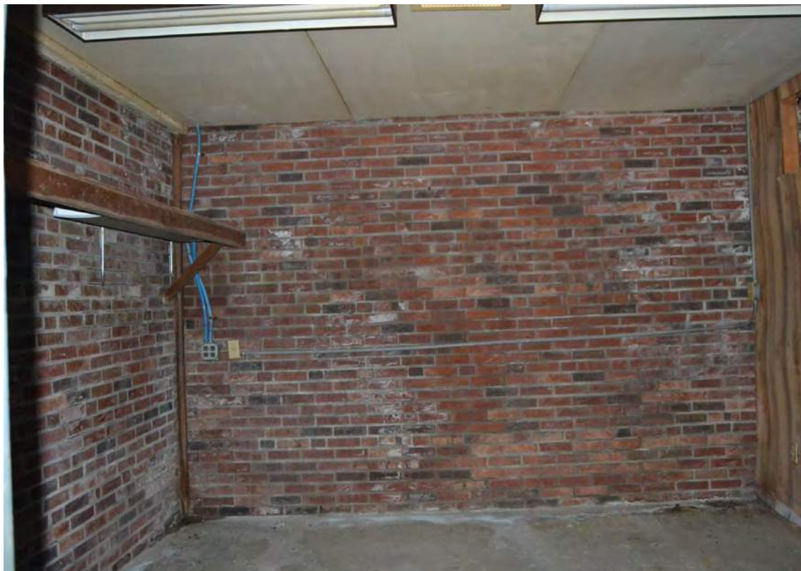
89. Grey Mill, 1970s Warehouse, Looking East
