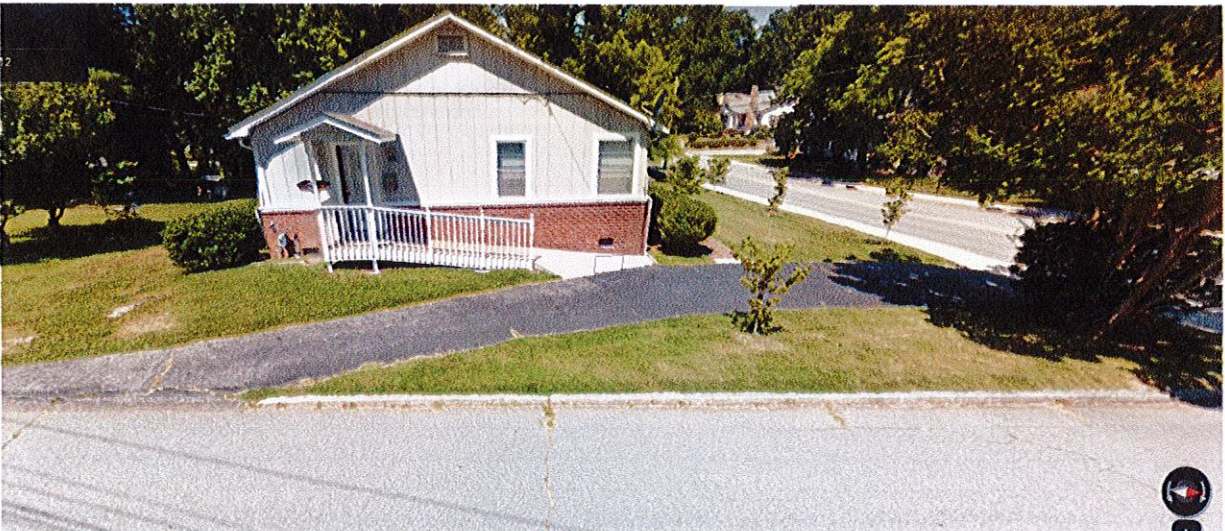
June 2012 -prior to the sale of the house in 2019 and subsequent removal due to deterioration and water damage.
