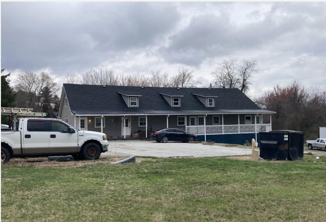
View of 5-unit multi-family structure on subject property (Hope Creek Ln.)
