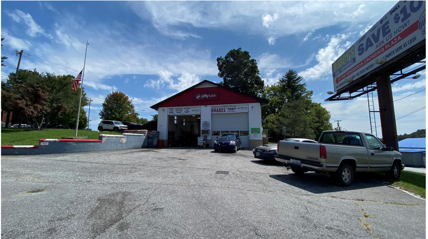
a.) Building Front
