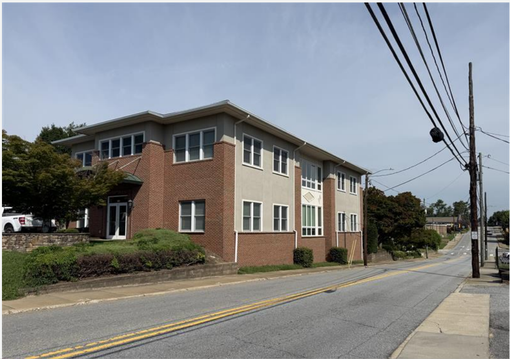
View of existing commercial building on the southern parcel from S Grove St.
