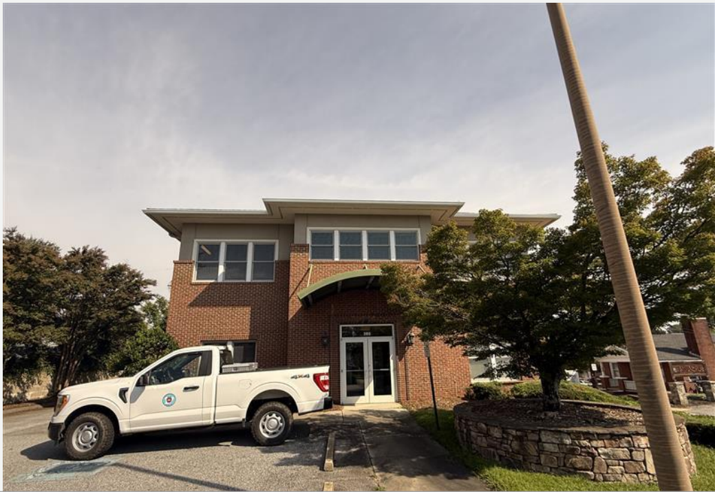
View of existing commercial building from the parking lot of E Allen St.
