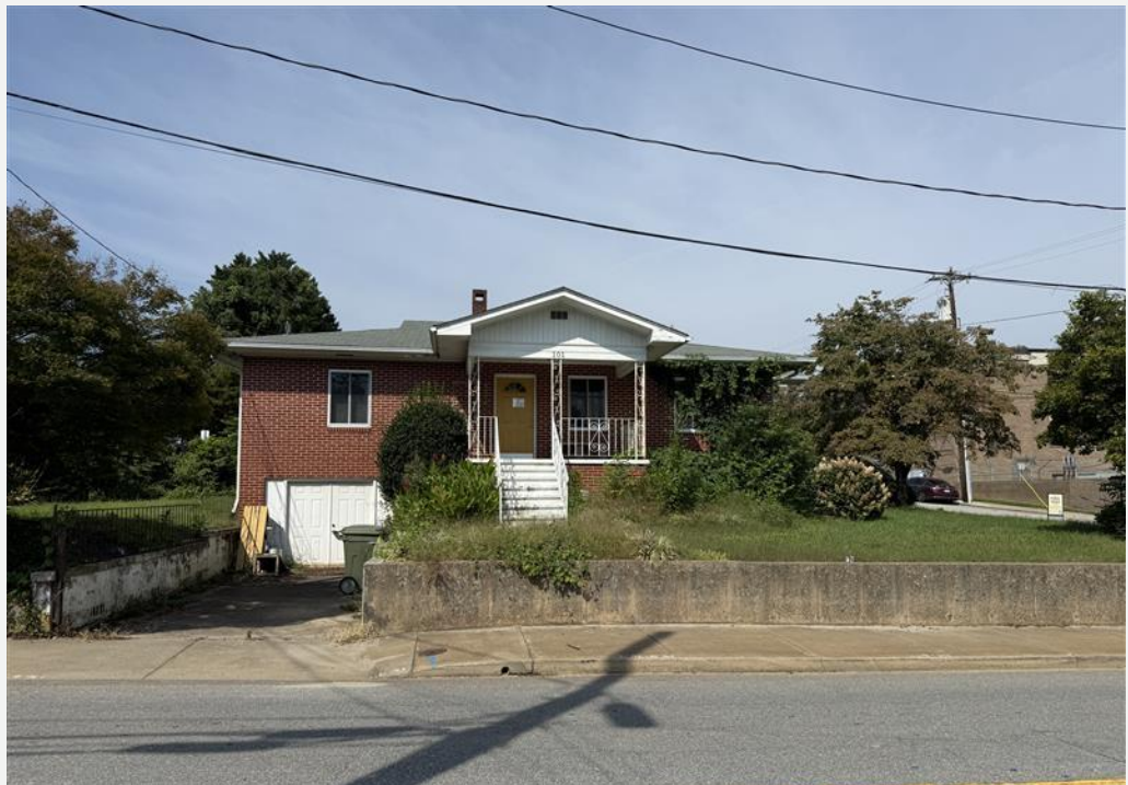
View existing house from S Grove St.
