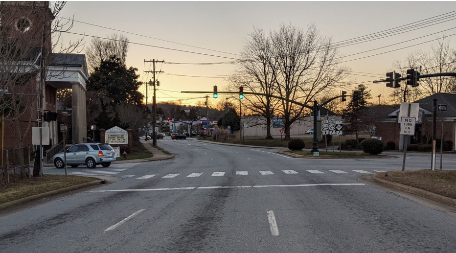
Photo of the intersection of 7th Avenue at Grove Street taken from the eastern approach. The skewed intersection increases the crossing distance and makes it more difficult to navigate for pedestrians.
