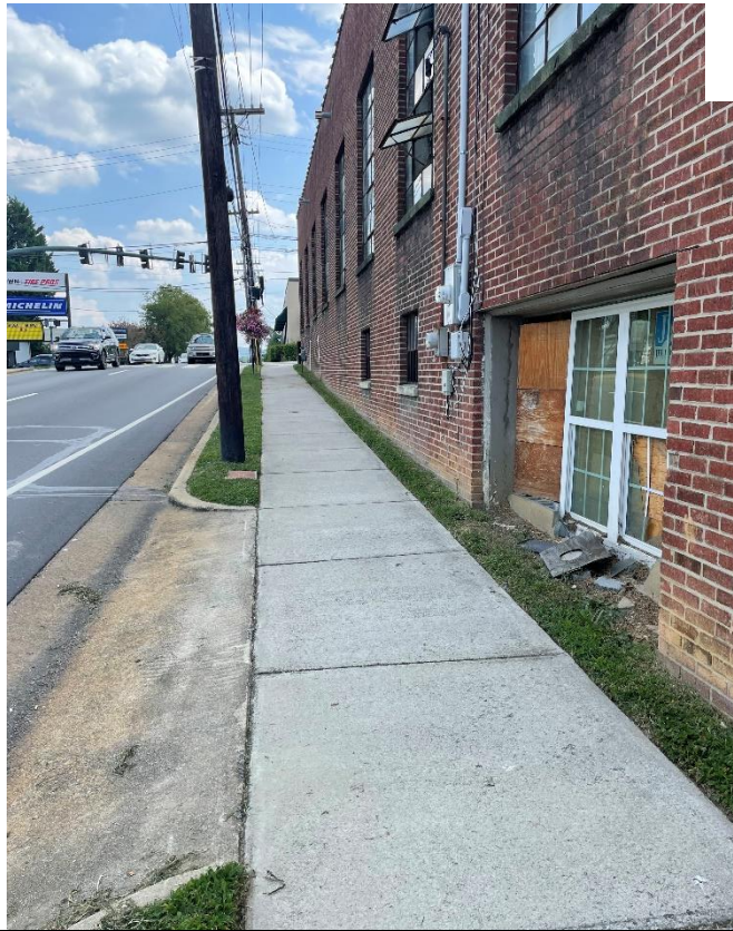
View of the curb cut, on King Street. Due to the curb cut, it appears that the building opening used to be some form of loading zone or entrance into the building.
