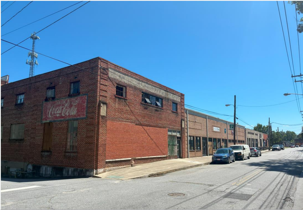
View of subject properties along Locust St that have been identified for potential rezoning
