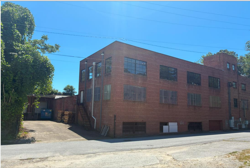
View of Side / Rear of previously rezoned property
