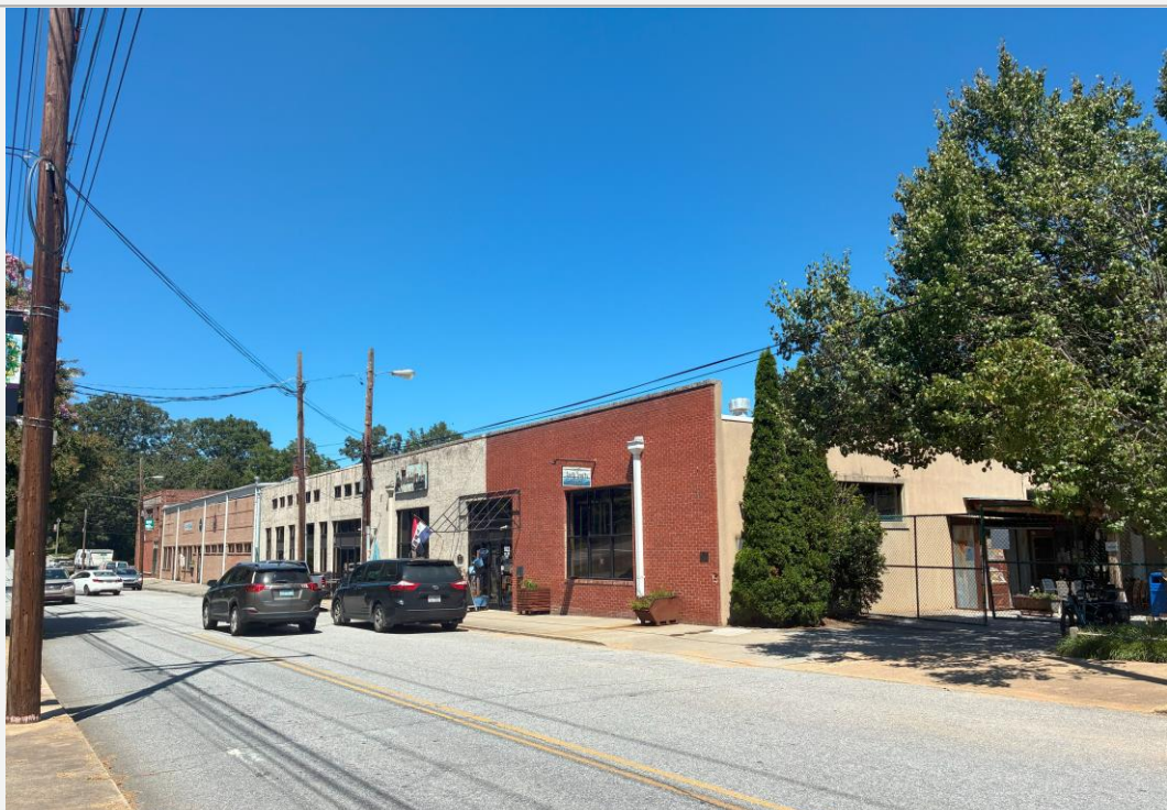
View of block of subject properties with buildings fronting Locust St that have been identified for potential rezoning
