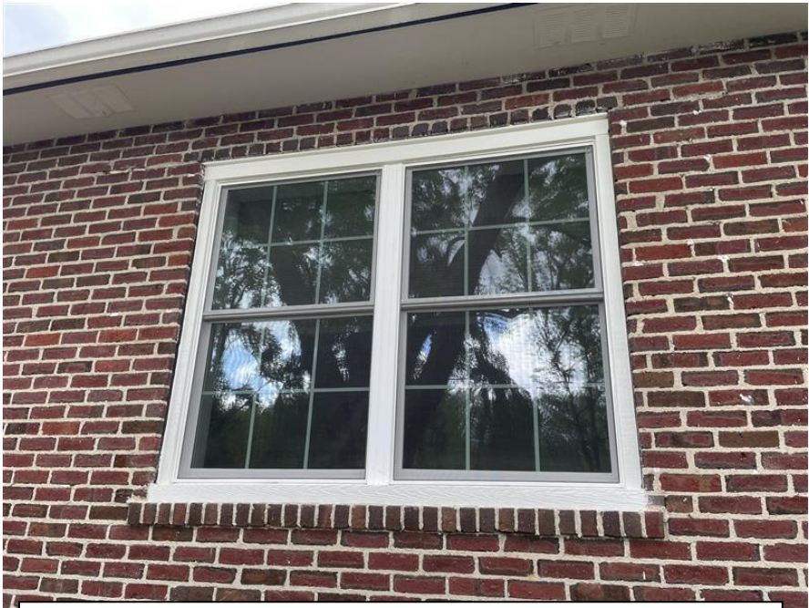
Windows located on southern facade. Photo provided by Staff.
