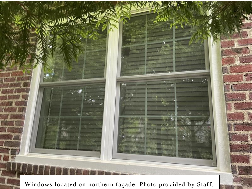
Windows located on northern façade. Photo provided by Staff.
