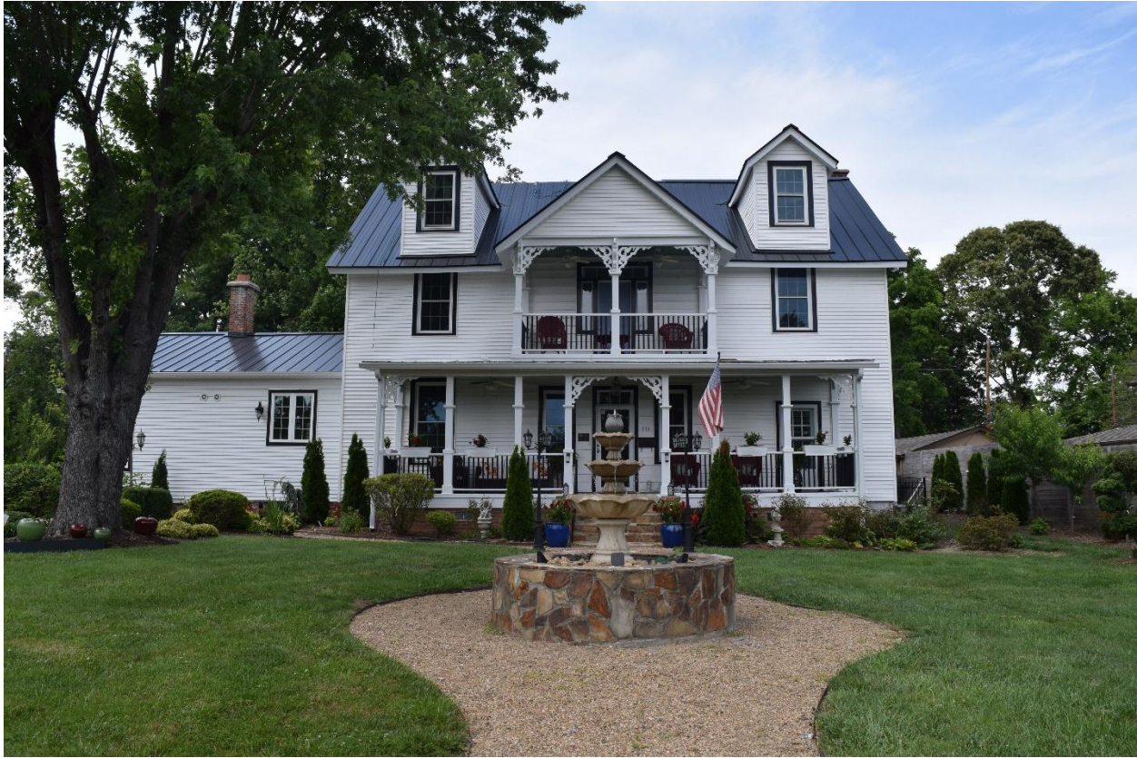
4. Front of house, view north
