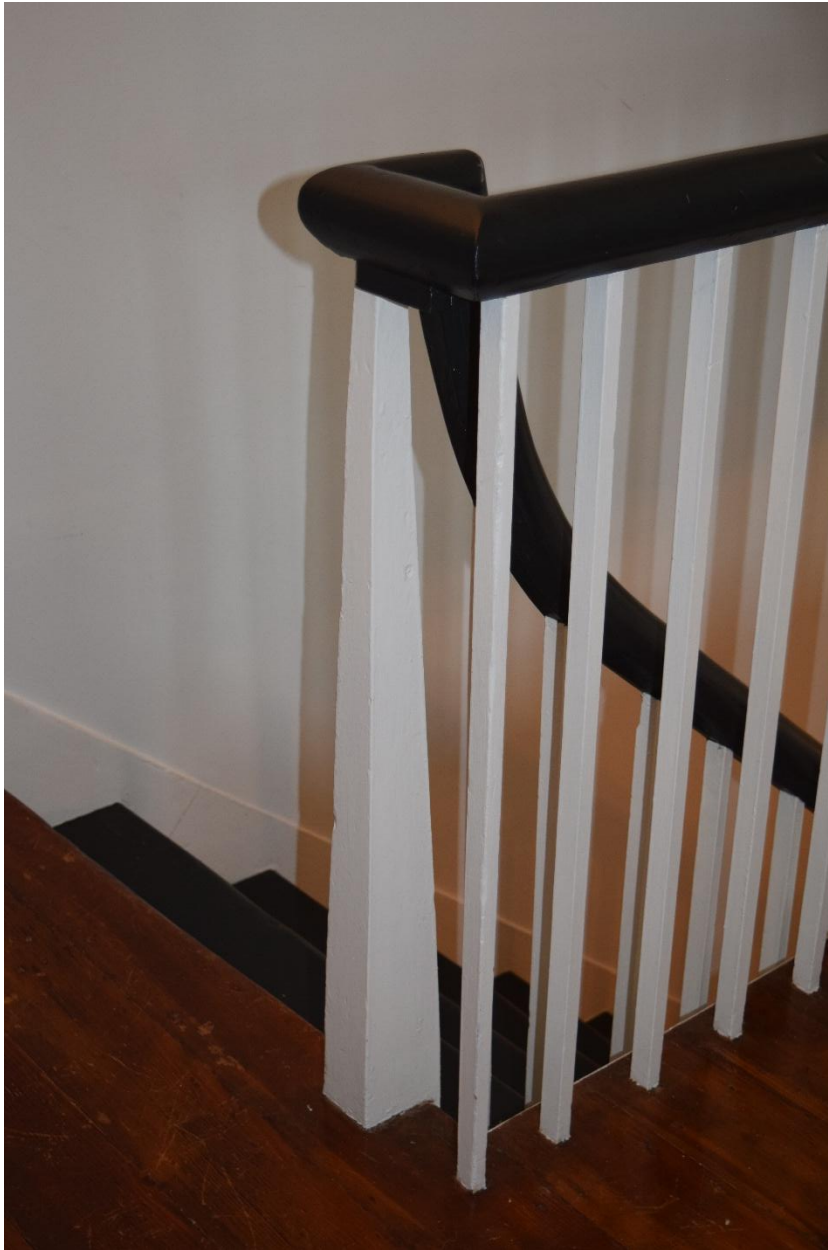
57. Second floor newel post and balustrade detail
