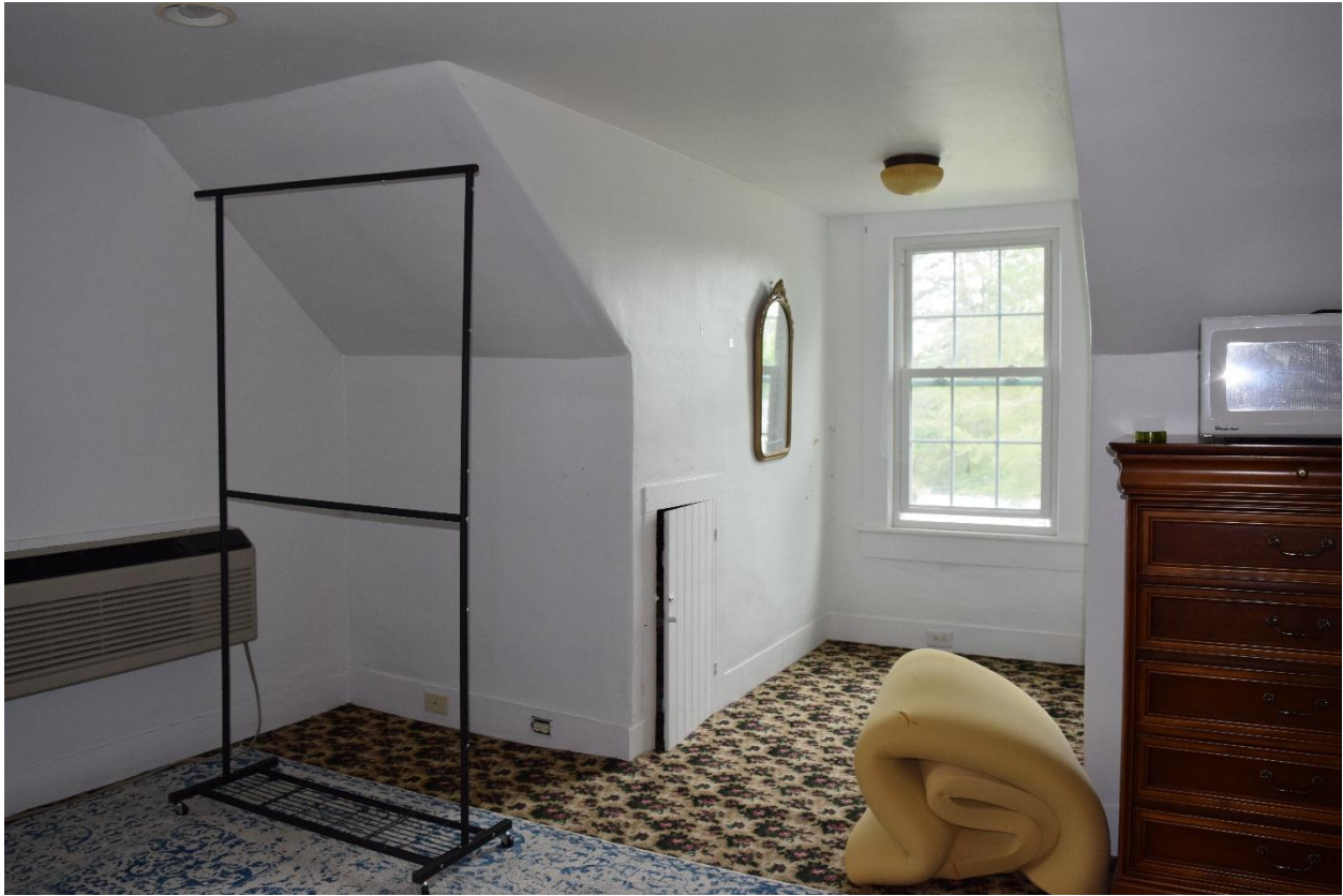
75. Attic storage, view southeast
