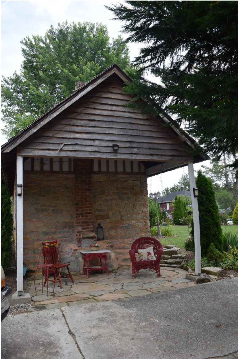
15. West elevation, carriage repair stone outbuilding, view southeast
