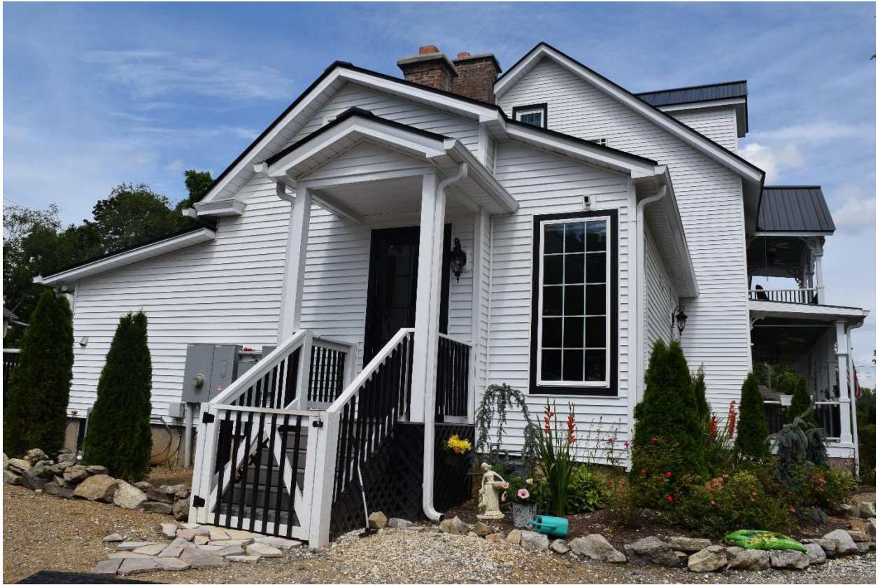
10. West elevation, kitchen wing, view northeast
