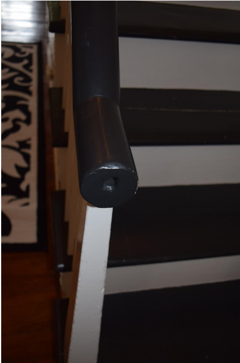
41. Banister detail, first floor staircase
