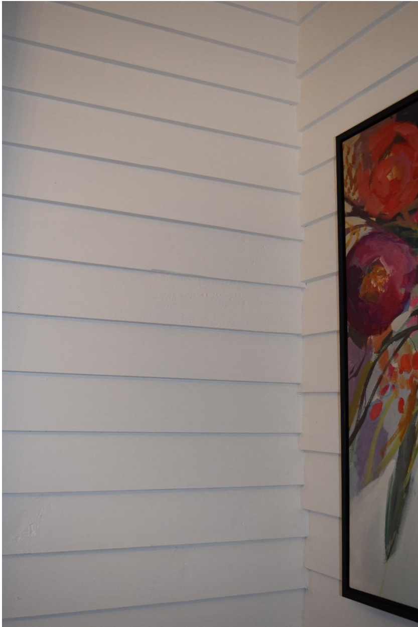
55. Second floor sitting room, south wall siding later infill
