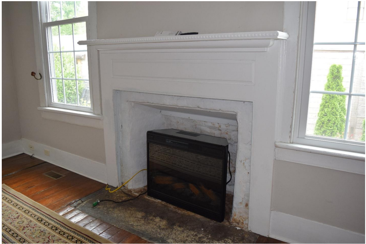
29. First floor bedroom mantel
