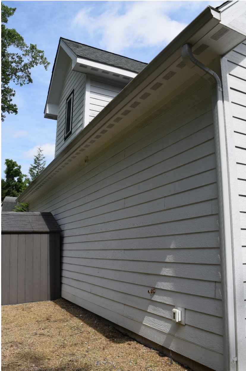
20. Non-historic garage, north elevation, view southeast
