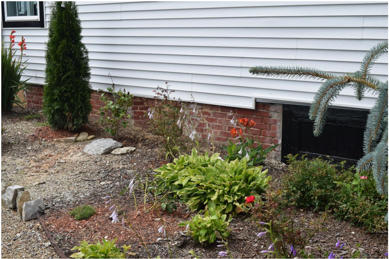
9. Brick foundation beneath kitchen wing, view northwest
