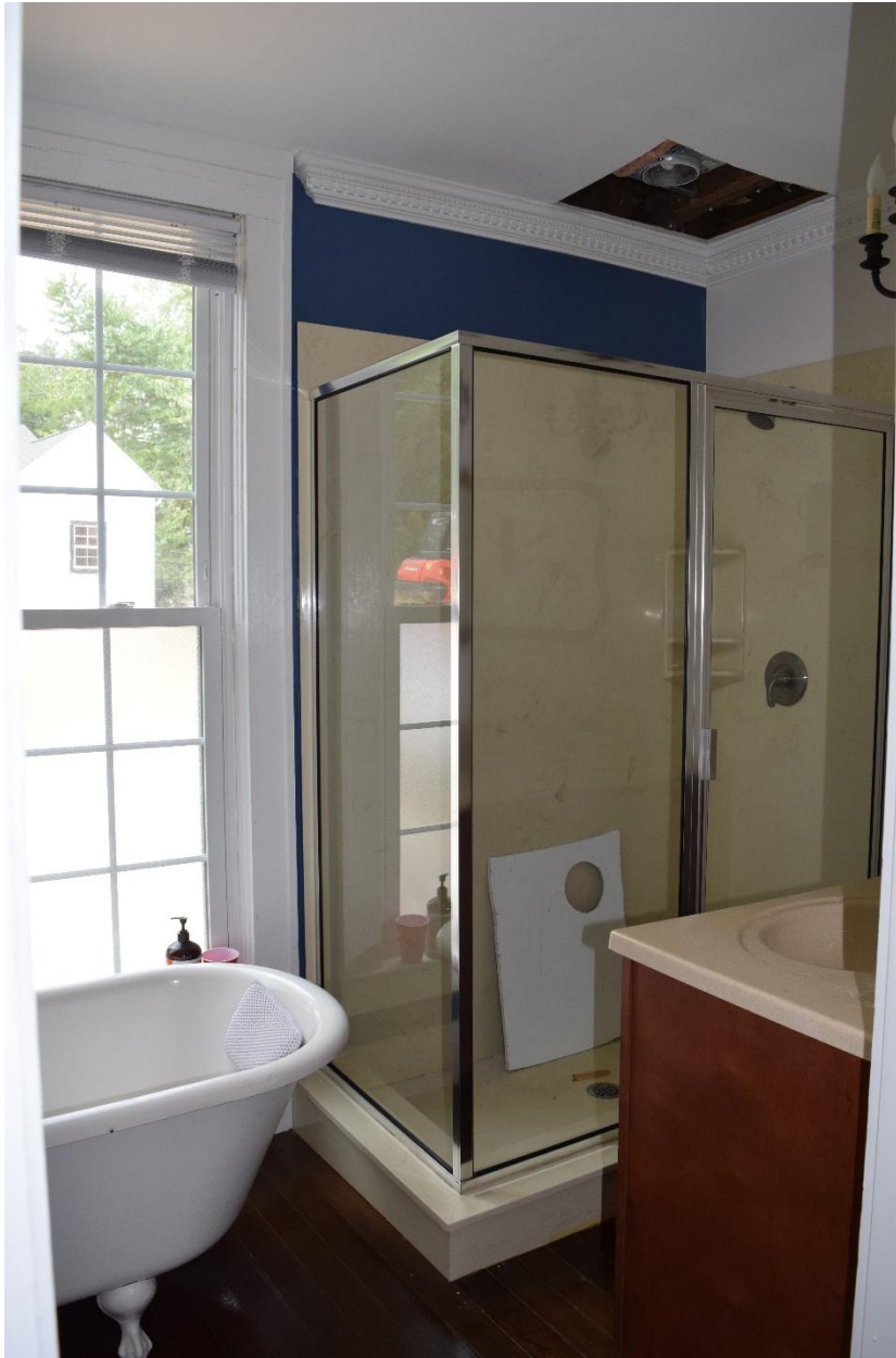
31. First floor bath, view northeast
