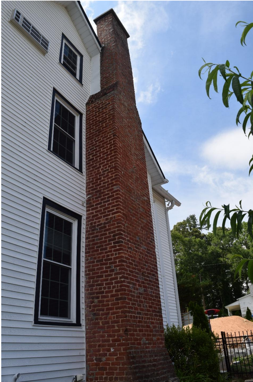
7. East elevation, single shoulder brick chimney
