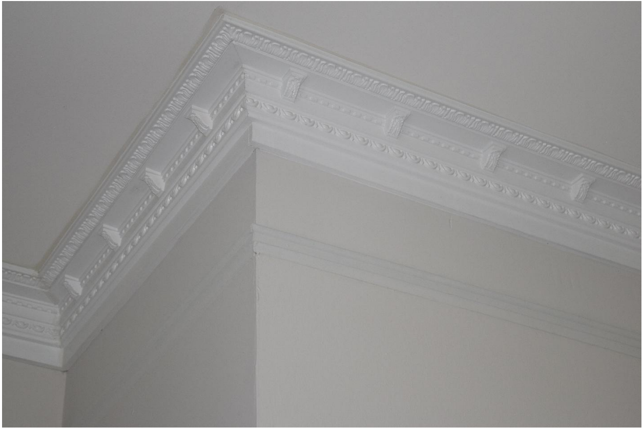
34. First floor crown molding
