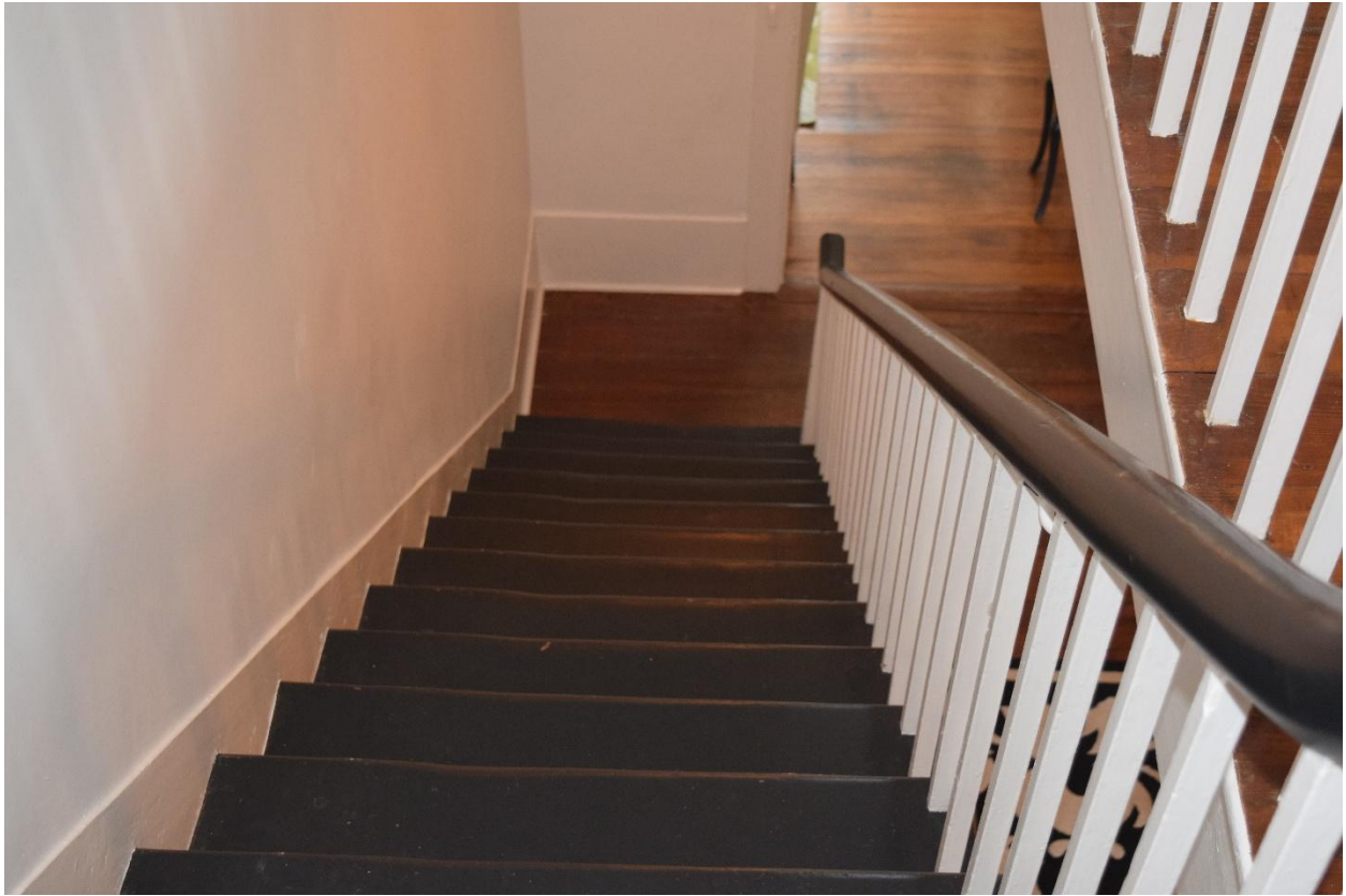
58. Staircase to first floor, view north
