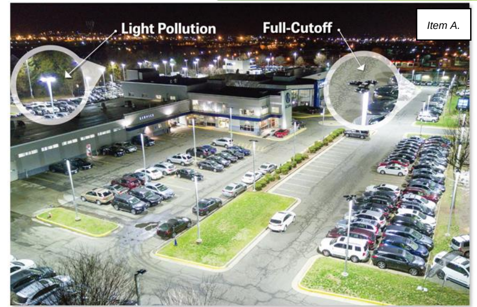
The retrofit on the front lot is completed while the rear lot has the original metal halide fixtures. Note the front lot LED lighting has no uplight from their full-cutoff, dark-sky compliant fixtures while the metal halide fixtures in the rear lot are light-polluting due to the substantial uplight
