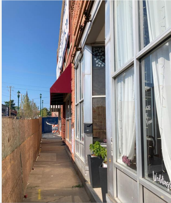
View along 7 th Ave facing southwest
