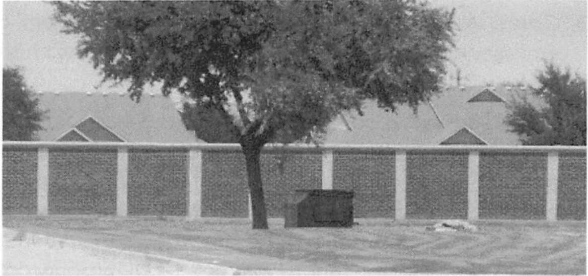
Eight (8') Foot Masonry Screening Wall
