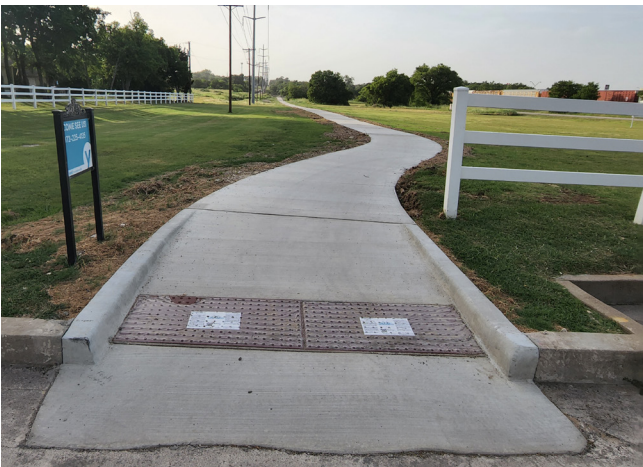
An existing trail connects Old Town to Campbell Park. A Trails Assessment would identify other potential trail connections in the community.
