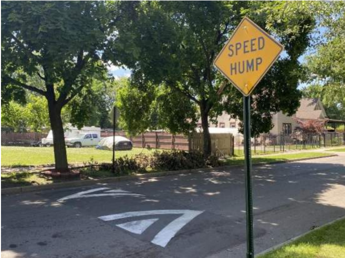
Figure 4: Speed Humps with Associated Signage
