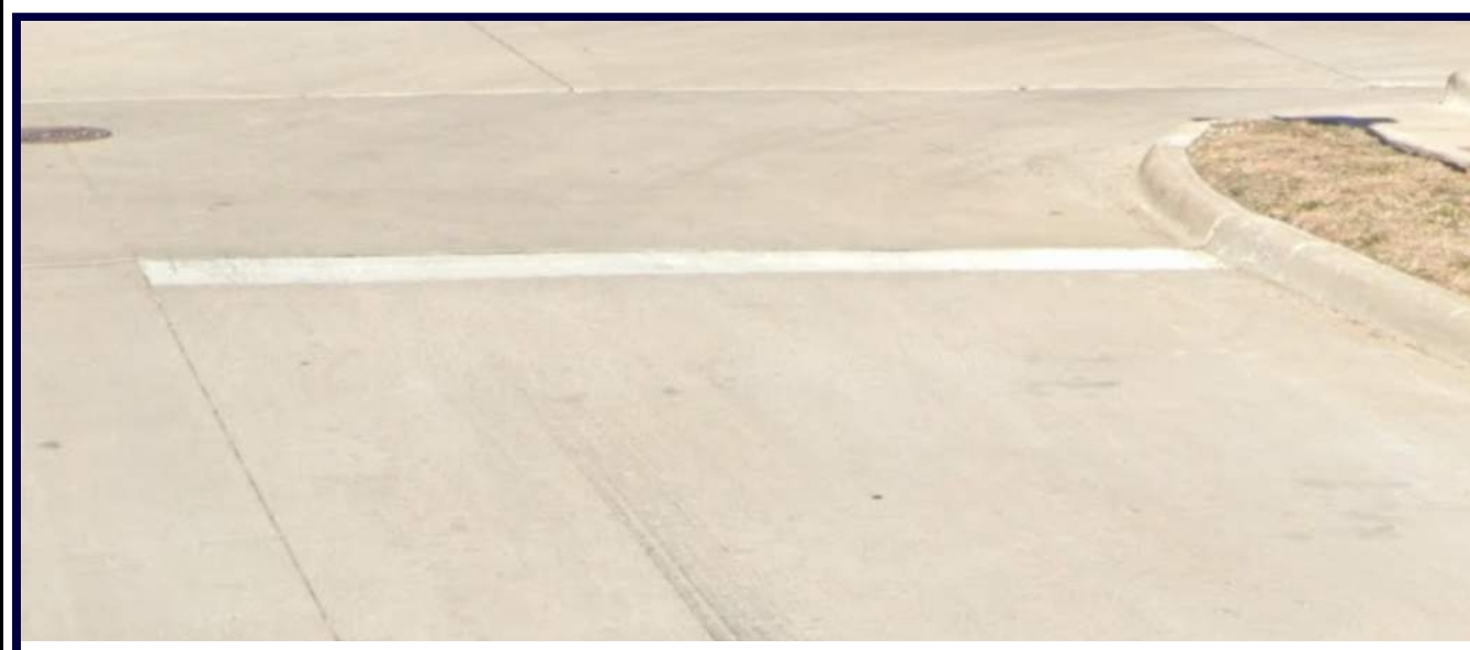
Install Stop Bar
