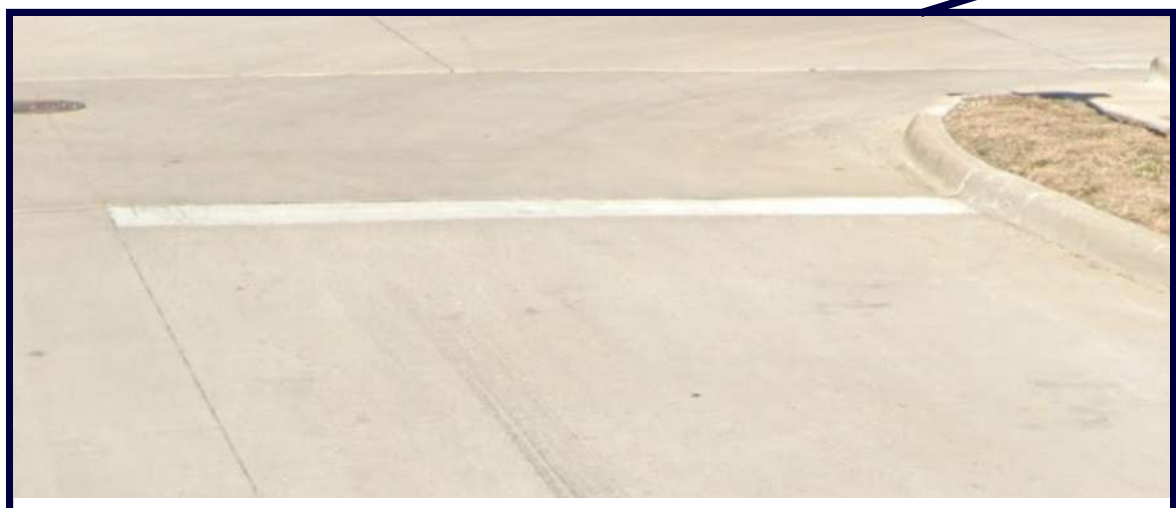
Install Stop Bar
