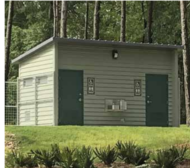
Flush restroom with custom roof pitch
