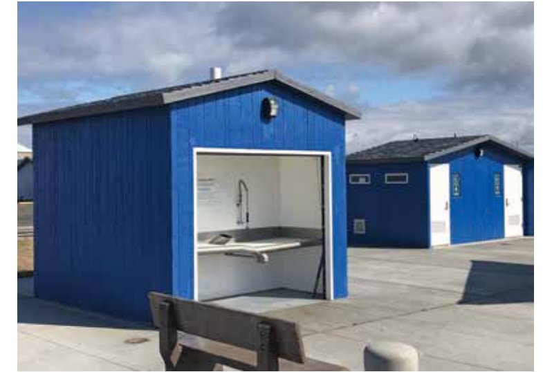
Flush restroom and fish cleaning station
