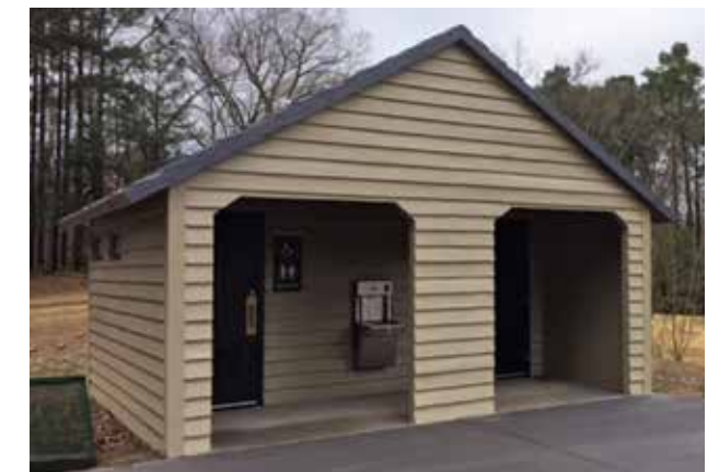
Flush restroom with golf cart shelter
