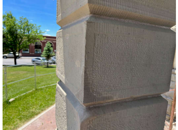
Photo #5: A corner of the entry porch column was patched with the tooling approved. Jahn mortar matching the stone will be provided.
