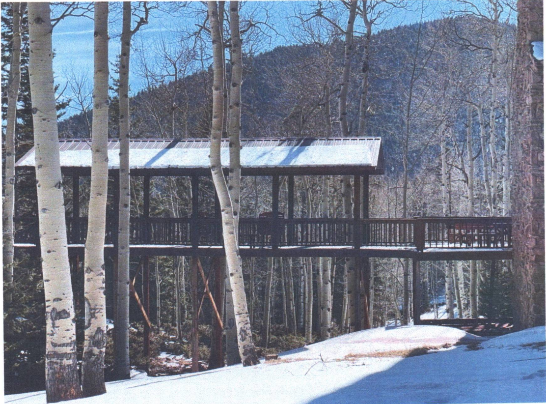
Example – McCombs bridge.
