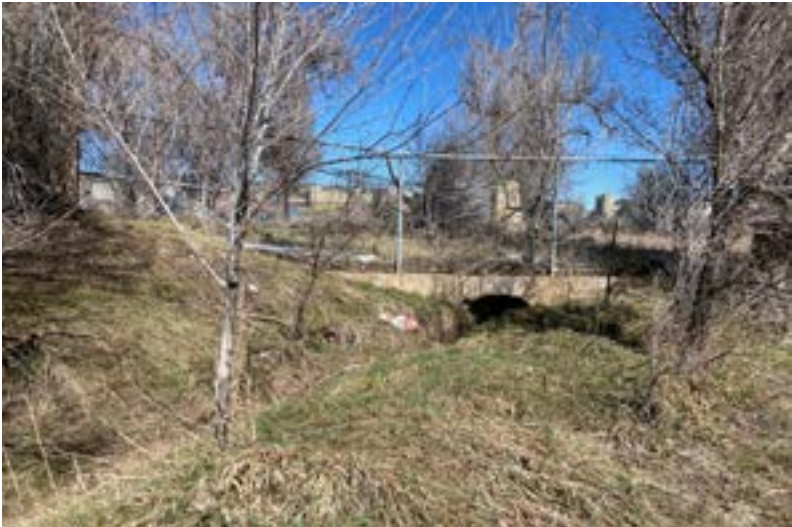
Irrigation ditch on northwest side of property
