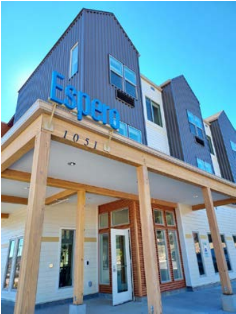
SW Housing Solutions Former Football Field
