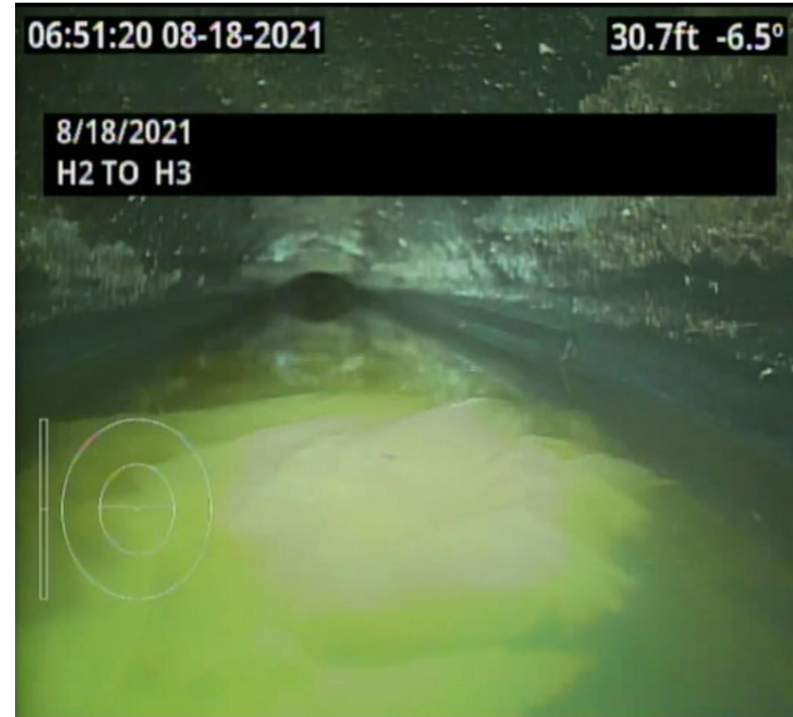
Sag between MH-H2 to MH-H3
