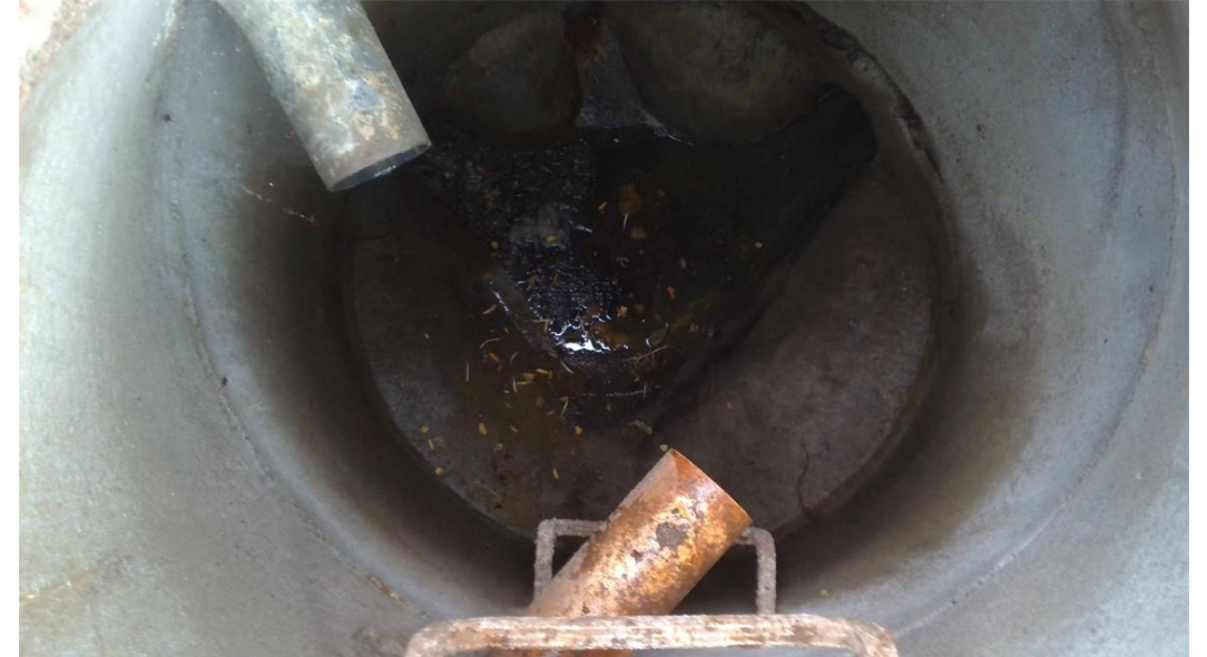
MH-14B- Service lines into manhole
