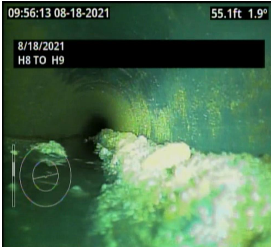
Debris between MH-H8 to MH-H9
