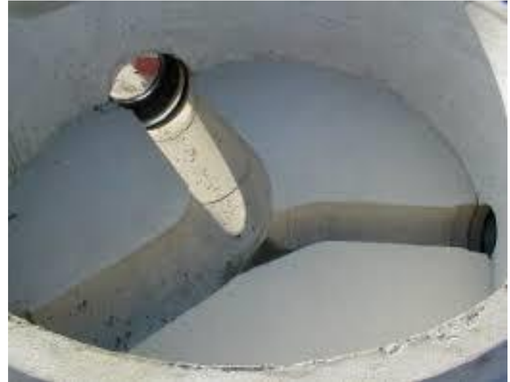
Picture of a new manhole base
