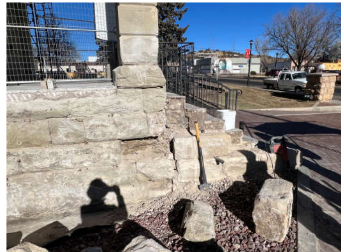
Photo #2: East end of south cheek wall showing deteriorated condition of original sandstone.
