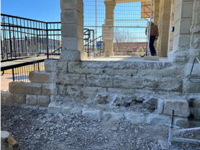
Photo #3: East end of north cheek wall with exposed original sandstone.
