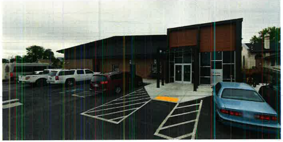
Exterior Exterior Rear VIEW OF REAR
