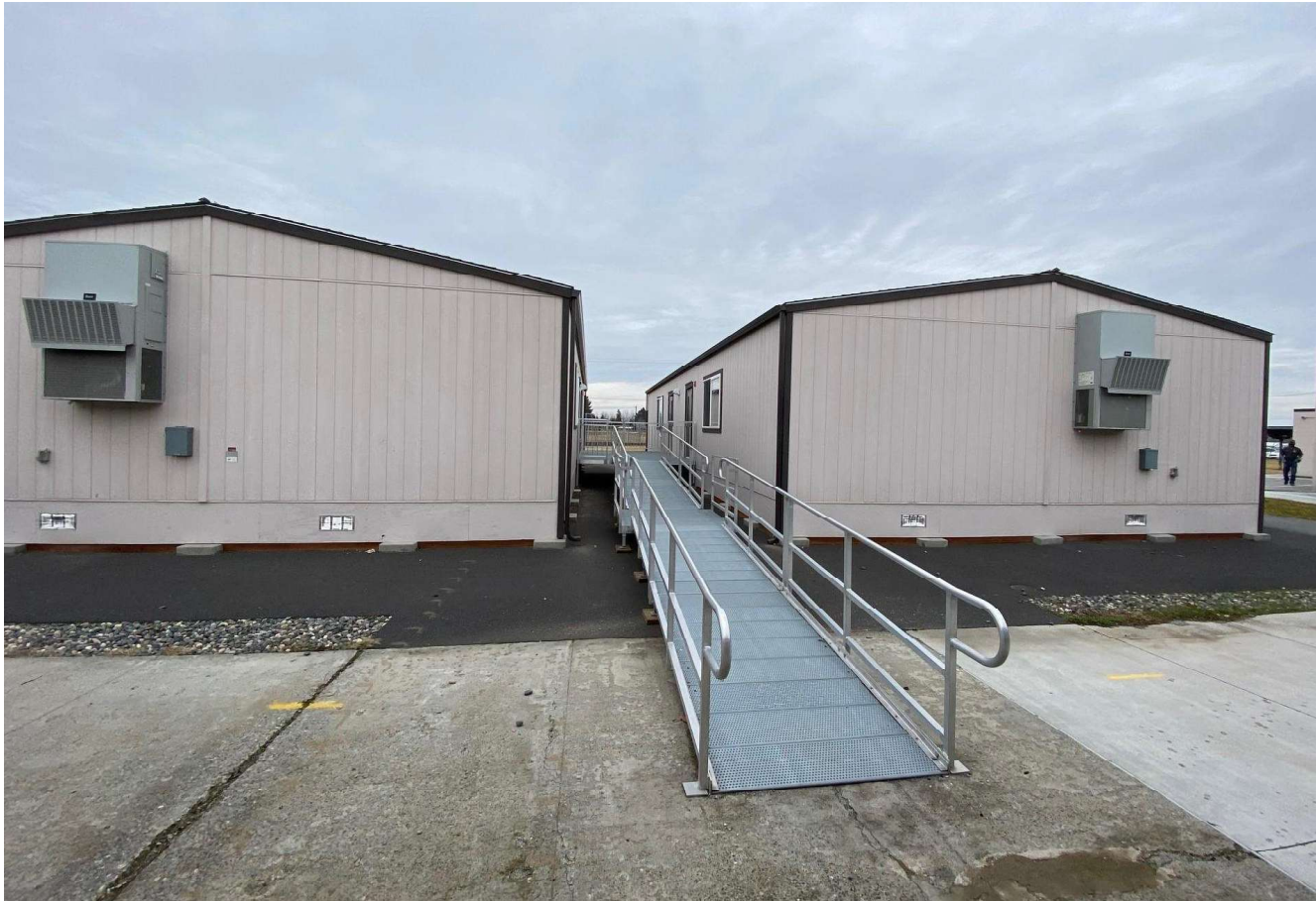
Existing portable buildings to be relocated. Currently located on Rocky Heights Elementary School site.
