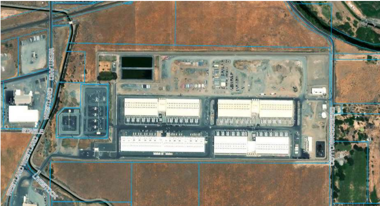
Figure 1: AWS Data Center, Umatilla County, Oregon Image Source: Umatilla County Interactive Map
