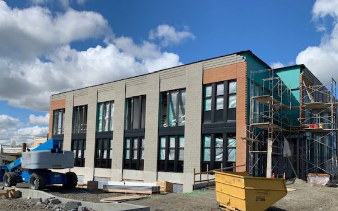
New City Hall Under Construction
