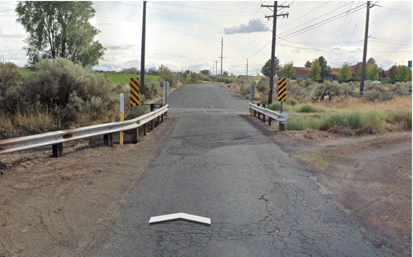
Southbound canal crossing
