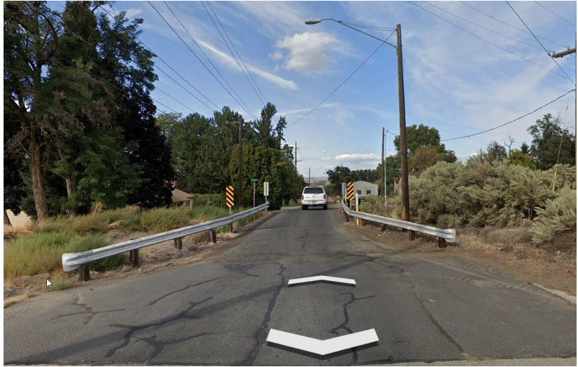
Northbound canal crossing
