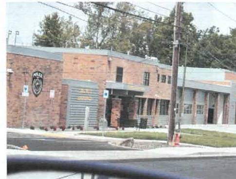
Public Safety Center
