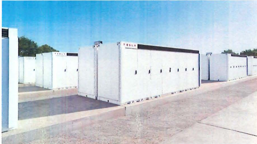
Figure 3. Tesla Battery Energy Storage System (BESS)
