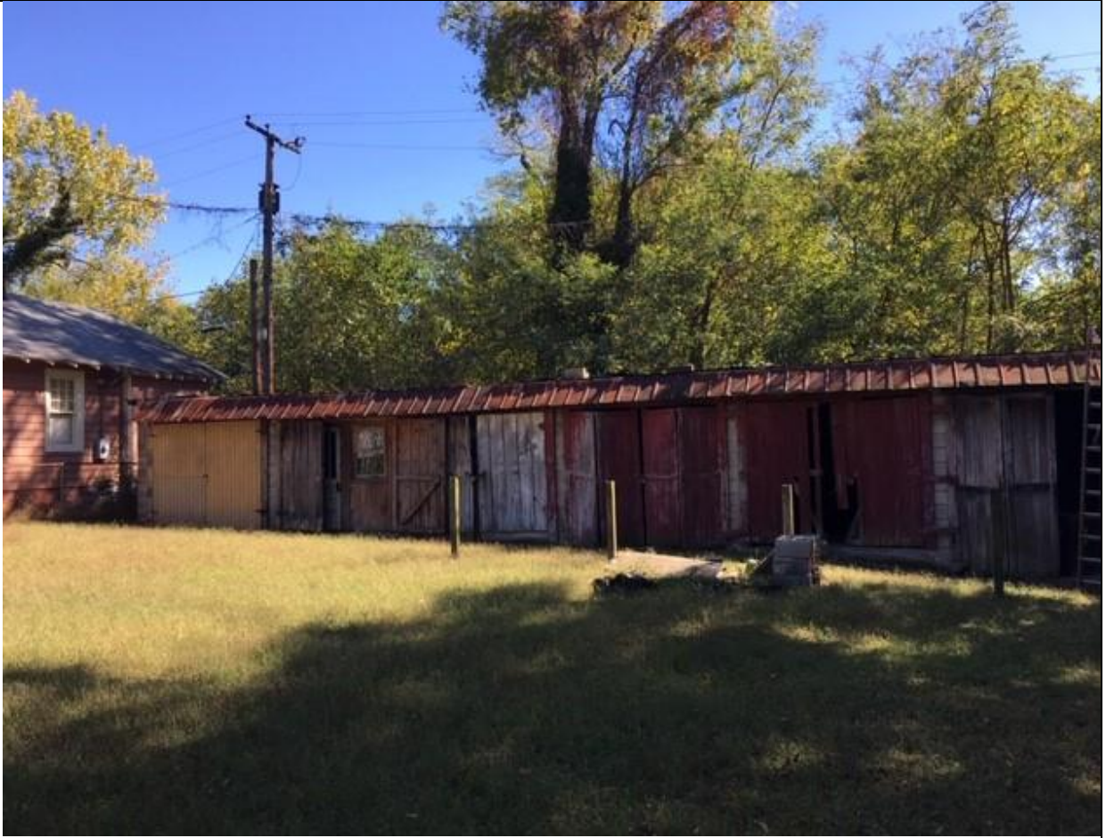
Metal garage structures
