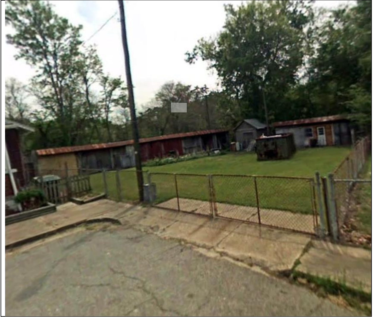
Street Level View of Garages
