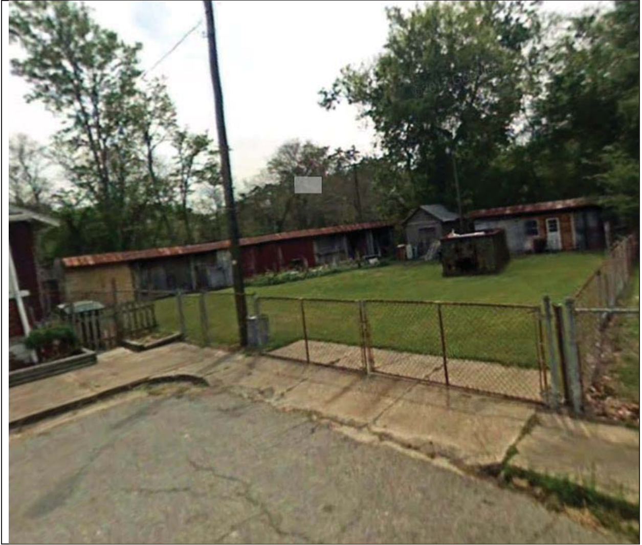
Street Level View of Garages
