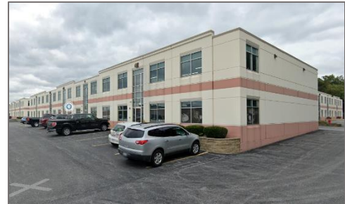
Figure 1: View of one building at the Homewood Business Park Condominiums complex @ 17759-17845 Bretz Drive.
