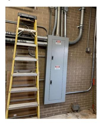
Figure 9 - Generator Distribution Panel
