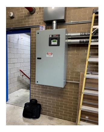
Figure 8 - Generator Automatic Transfer Switch
