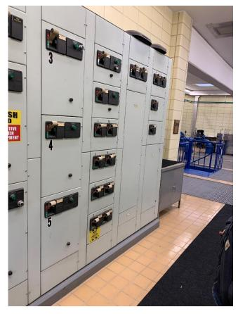
Figure No. 16 - Pump Station No. 1 Main Switchboard
