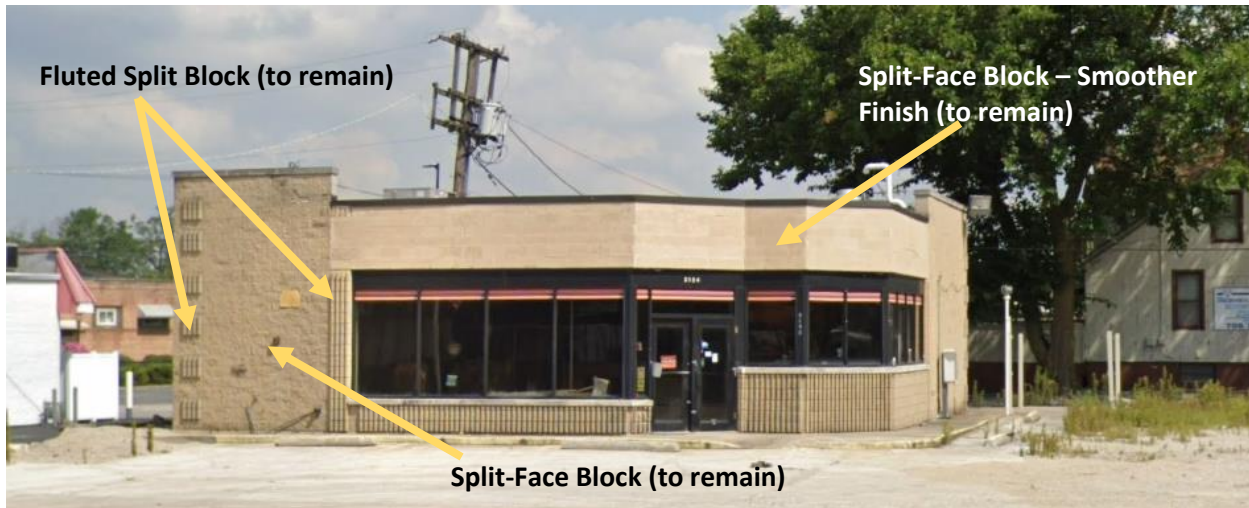
Figure 2: Existing structure on the site with materials identified. Plans for use of materials in redevelopment identified on image.
