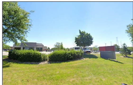
Figure 1: Existing building as of June 2024, including MOD Pizza exterior renovations.
