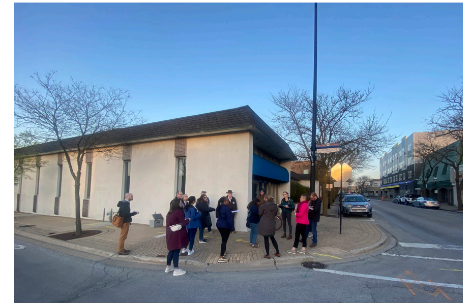
Fig. 23. Site from the Southwest
