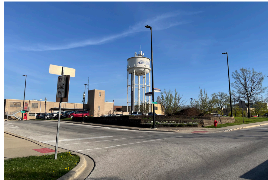
Fig. 21. Site from the Northwest
