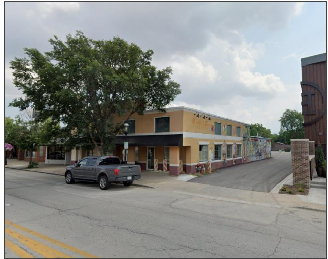
Figure 1: The existing building located at 18219 Dixie Highway (former Mama and Me Pizzeria)
