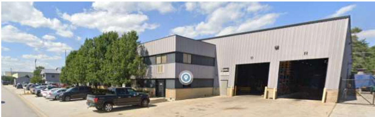
North side of 175 th St. across from the Project Site
