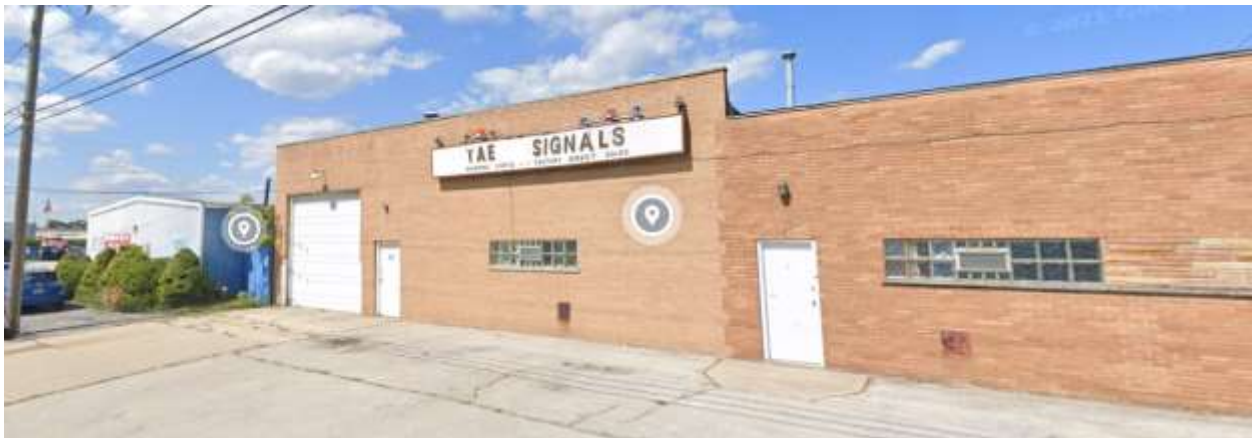
T.A.E. Signal located at 1516 175 th St. (west of the Project Site on the north side of 175 th St.)
