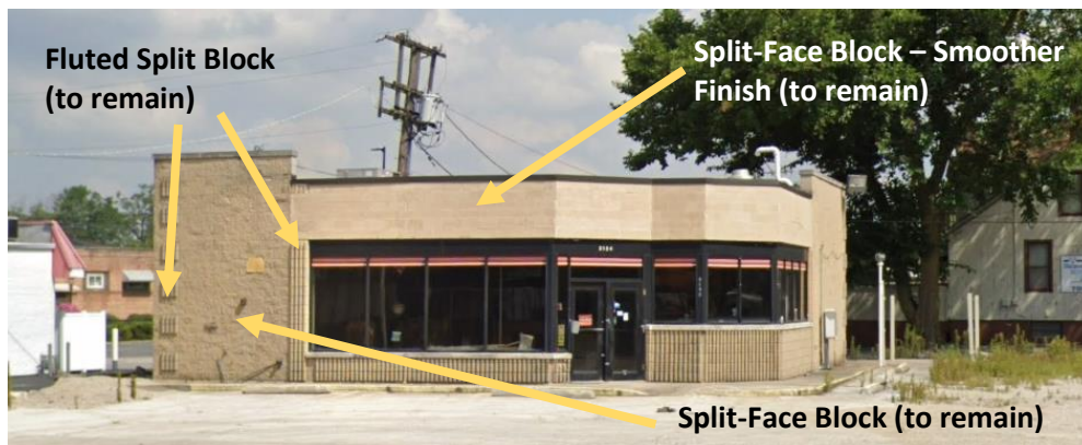
Figure 1: Existing structure on the site with materials identified. Plans for use of materials in redevelopment identified on image.
