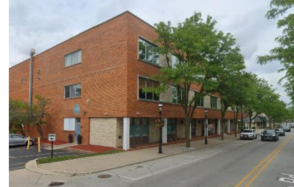
Figure 1: Golden Eagle Office Center in 2025
