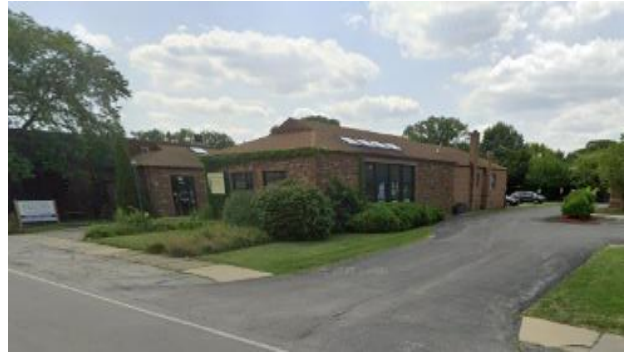
Figure 1: Image of current building frontage at 18646 Dixie Highway
