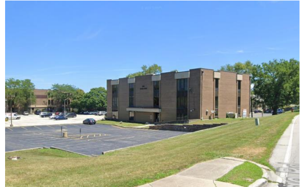
Figure 1: Location of proposed business, in an office building at 900 Ridge Road
