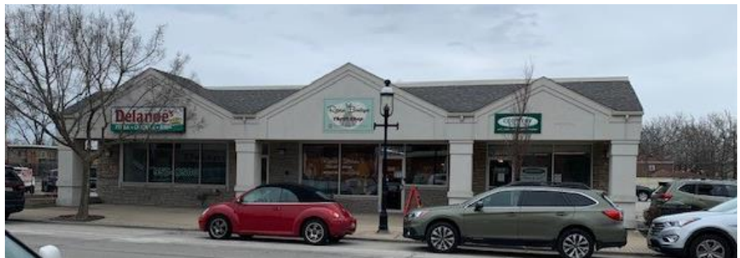
Subject property as viewed from Dixie Highway
