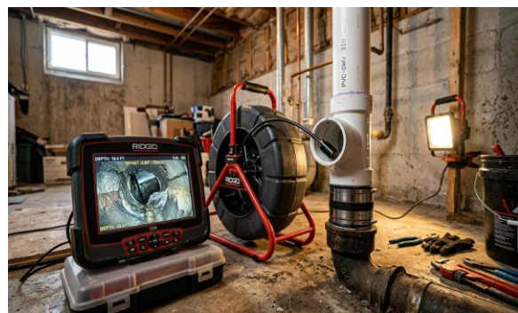
Televising a Sewer Cleanout
