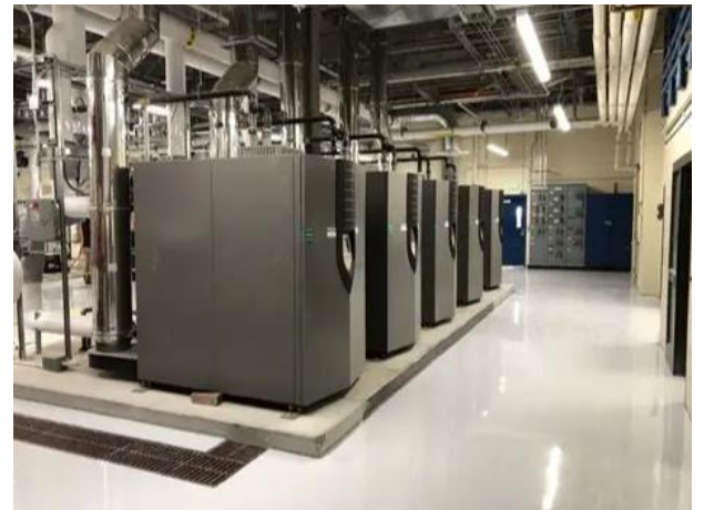
High-efficiency boilers
