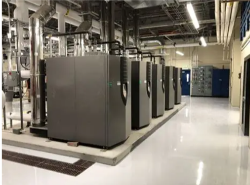
High-efficiency boilers
