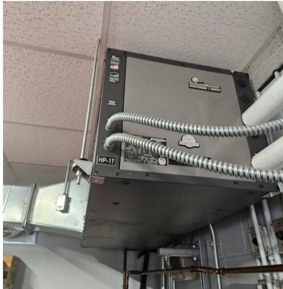
Typical ducted ground source heat pump
