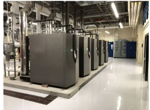
High-efficiency boilers
