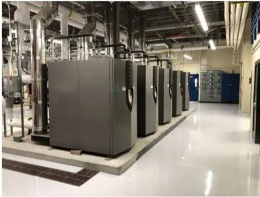
High-efficiency boilers
