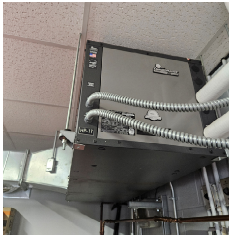
Typical ducted ground source heat pump
