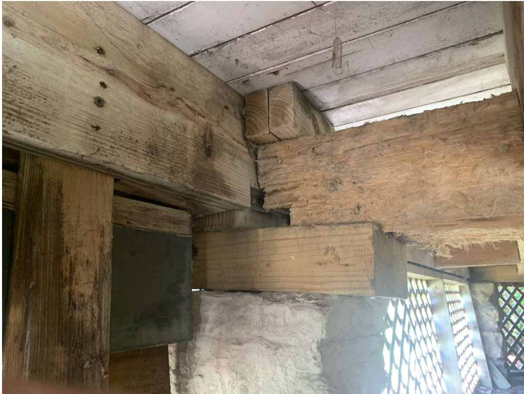
BEAM ON STONE PEDESTAL & BLOCKING
