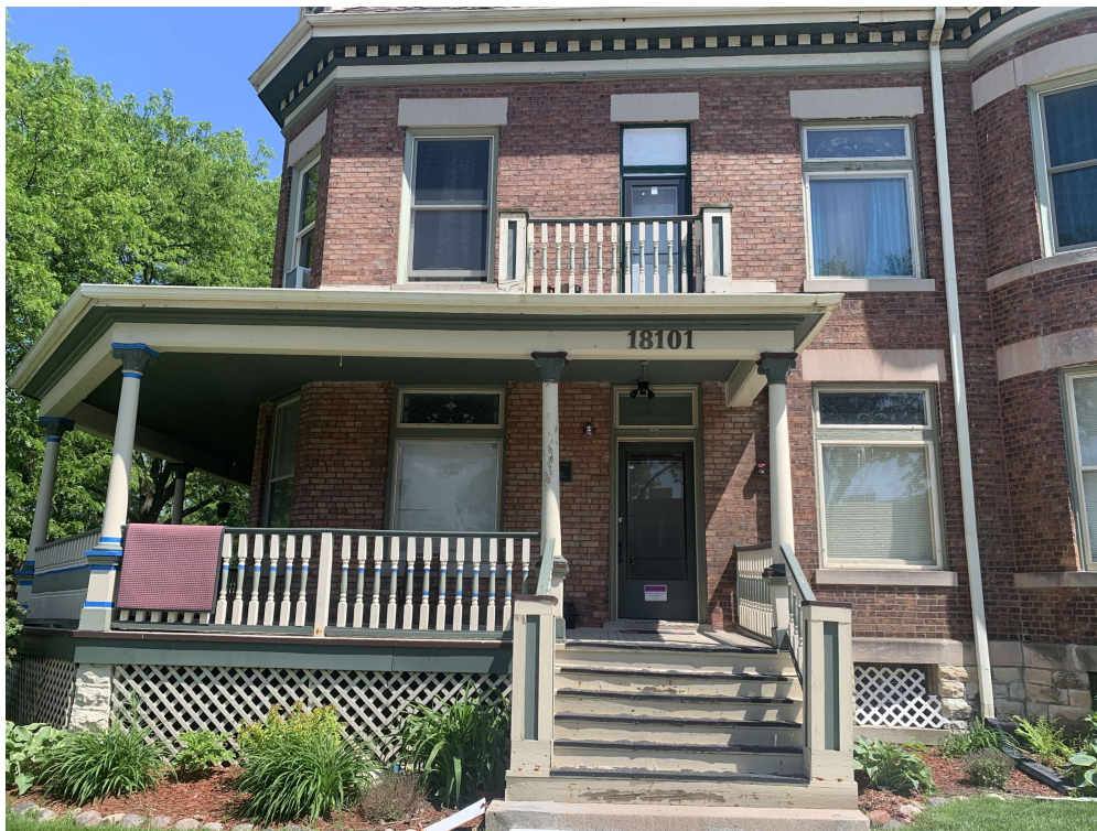
STREET VIEW OF FRONT PORCH
