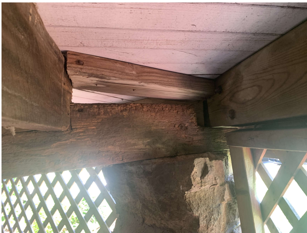
BEAM ON STONE PEDESTAL & BLOCKING
