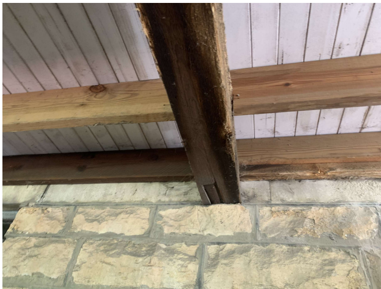
TYPICAL POCKETED BEAM & NOTCHED DECK JOISTS
