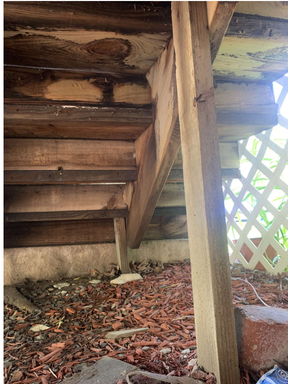
STAIR FLIGHT W/ POSTS ON GRADE
