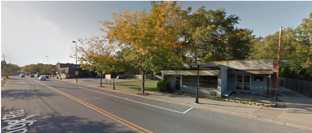
Figure 1: The appearance of the 1700 block of Ridge Road, prior to the demolition of most vacant structures on the site in 2017 (Source: Google Maps, 2013 imagery). The subject property is located in the foreground of the image.
