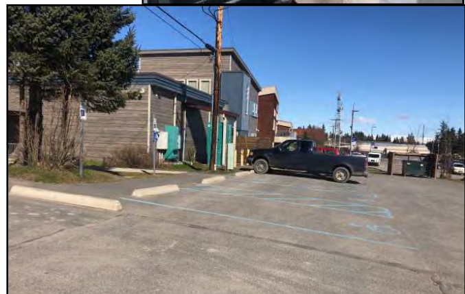
The cross slope of the accessible parking spaces at the lower entrance to City Hall exceeds the maximum allowed.
