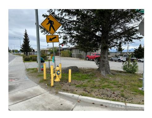
Large spruce tree at City Hall is preventing the replacement of a failed fire hydrant that requires replacement (not functional and not repairable)
