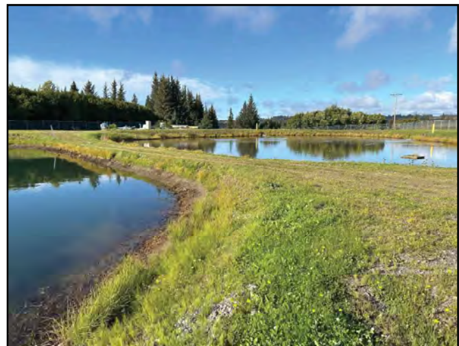
Particulate from the raw water filtration process settles in ponds at the Water Treatment Plant (above) before being removed to dry in beds (below) in preparation for transport to the landfill.
