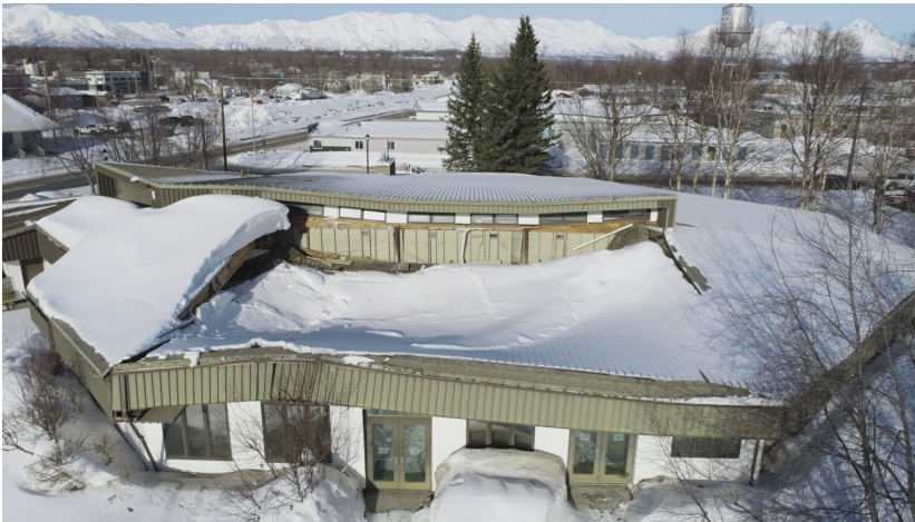
The roof on the Palmer Public Library partially collapsed on Feb. 15. (Courtesy PND Engineers)
