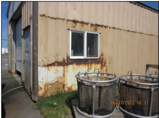
A new building made of corrosion-Resistant materials is compromising the Fish Grinding building's structural integrity and degrading interior fixtures.
